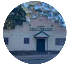
Existing community building (Former Scout Hall)
