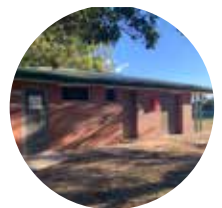
Existing amenities building
