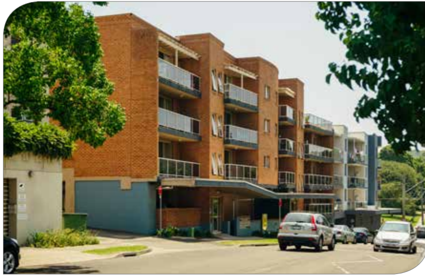
Victoria Road East Precinct, viewing north from Anzac Avenue.
