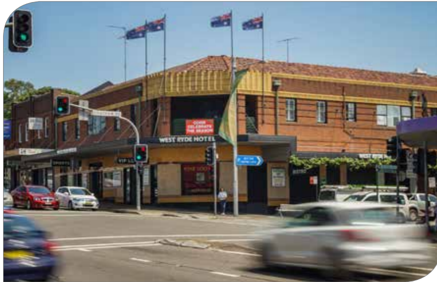
Victoria Road West Precinct, viewing northwest to West Ryde Hotel from the southern side of the Chatham Road intersection.
