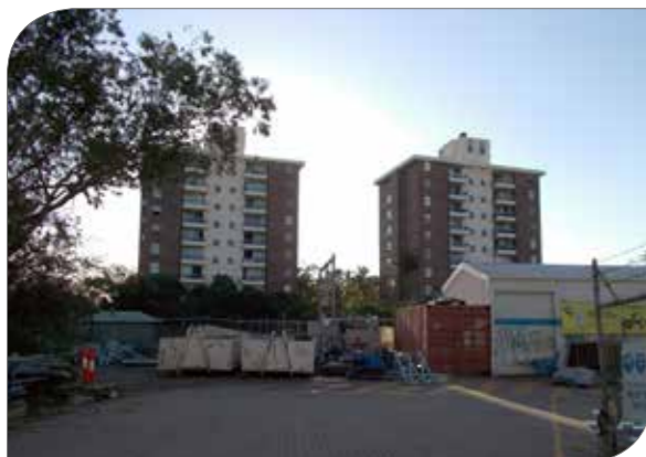
No. 57-61 West Parade, existing residential towers highly visible from surrounding areas and serves as a marker of West Ryde Town Centre.
