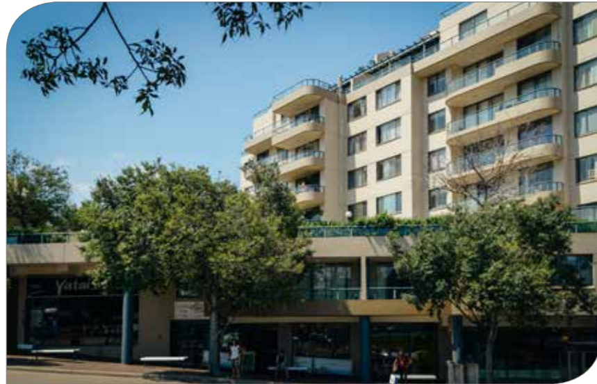
Station Precinct, viewing east to the existing development at 1-55 West Parade.
