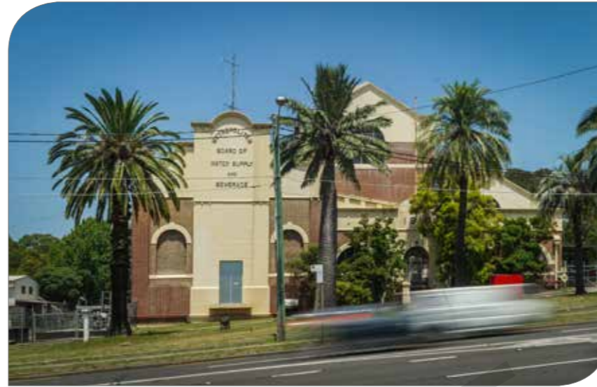
Pumping Station Precinct, viewing southeast from Victoria Road.
