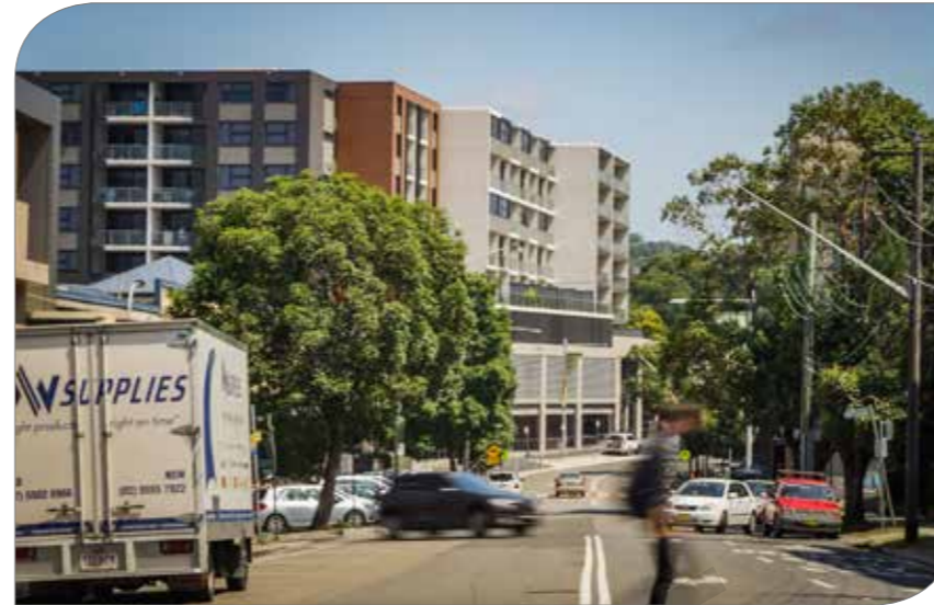
Town Centre Core Precinct, viewing northwest from Anthony Road.
