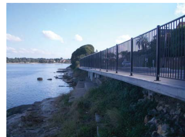
Precedent Image of Suspended Pavement Elevated concrete pavement on road verge to maintain consistent pathway widths. (Canada Bay Trail).
