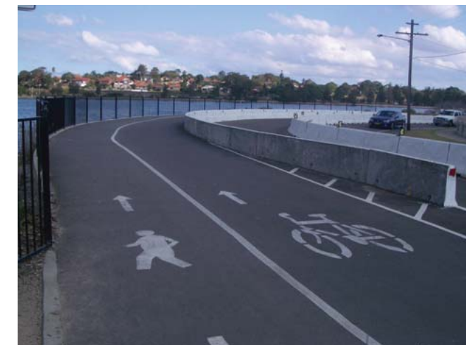
Precedent Image of Segregated Footpath Defined pedestrian and cycle lanes within path to reduce conflict in key areas. (Canada Bay Trail).
