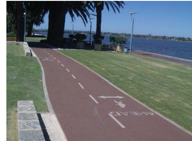
Precedent Image of Main Pathway Pathway used for commuting and recreation purposes with painted linemarkings (Swan River, Perth)
