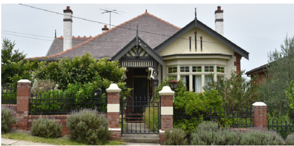
Have your say on protecting our local heritage and character in the City of Ryde.
