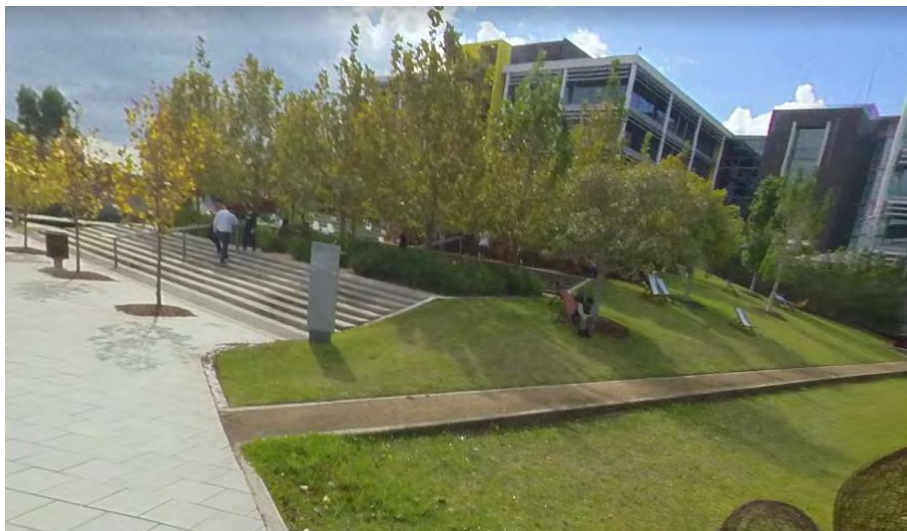
Figure 8: Photograph of stairs and trees to be removed/demolished.
