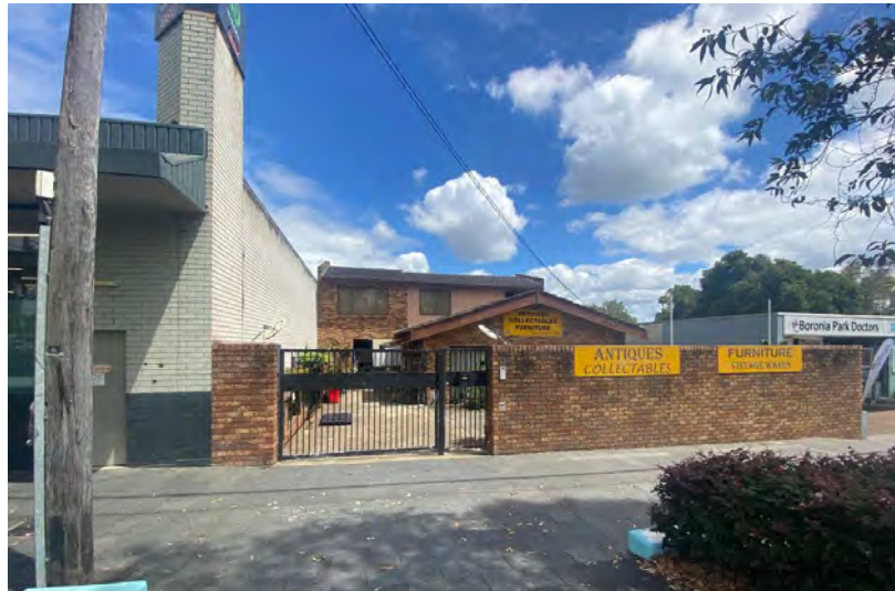
Figure 10: 136 Pittwater Road located within the centre of the image. To the right of frame is 138 Pittwater Road. Source: CPS – Site Inspection, 16 January 2023.
