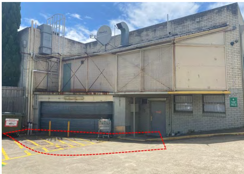
Figure 19: Location of depression identified in red & exhibits an existing ground level ranging from RL 47.38 to RL 47.79. Source: CPS – Site Inspection, 16 January 2023
