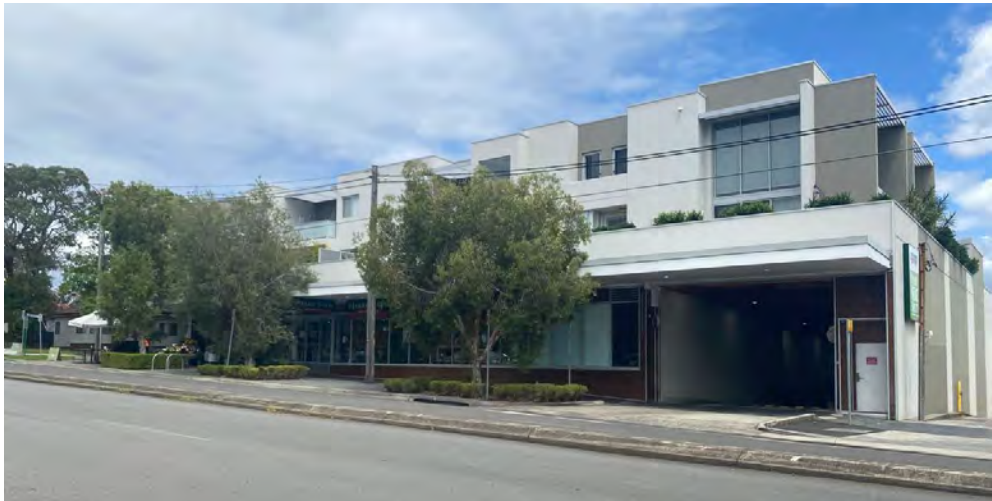
Figure 7: 126-128 Pittwater Road shop top housing development. Source: CPS – Site Inspection, 16 January 2023.
