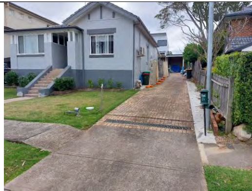
The existing dwelling and access handle as viewed from Spencer Street.
