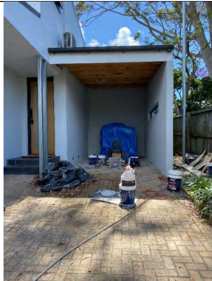
Existing car parking structure at 7A Spencer
