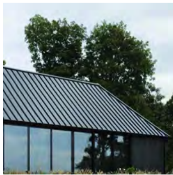
3A METAL DECK ROOF COLOUR: CHARCOAL GREY (COLORBOND MONUMENT OR SIMILAR)
