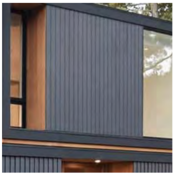
2 VERTICAL CLADDING EXPRESSED JOINTS COLOUR: CHARCOAL GREY
