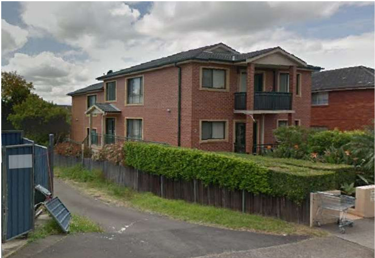
Figure 12: No. 2 Gowrie Street side elevation which faces the subject site.
