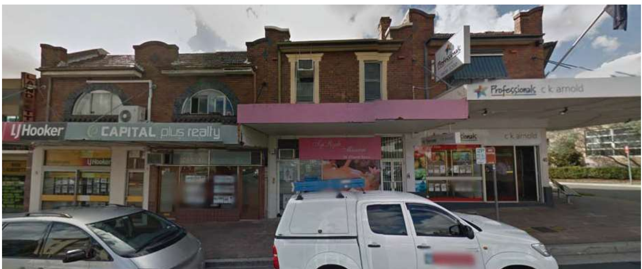
Figure 1: Church Street frontage of the site.
