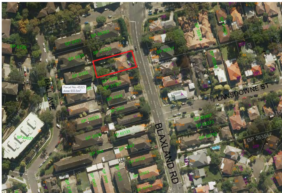
Figure 1: Aerial photograph of the site and surrounding area. Subject site outlined in red.
