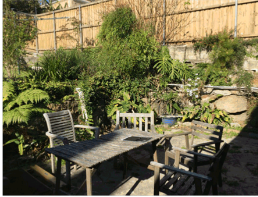
2318 - Patio at front of dwelling, view east to area of excavation for additions
