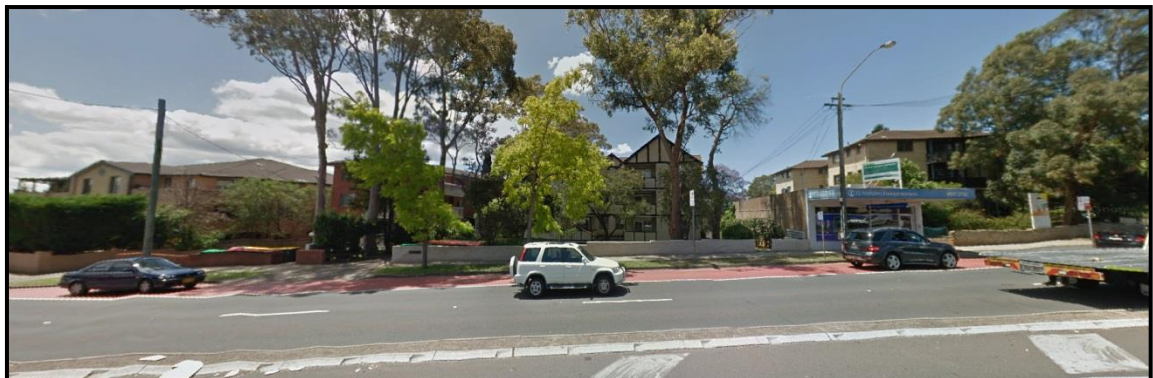
Figure 6: Streetscape character of Victoria Road
