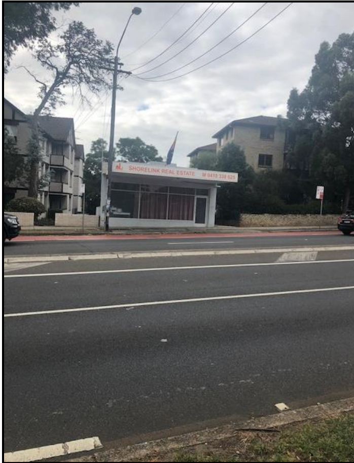
Figure 2: Victoria Road frontage of the site
