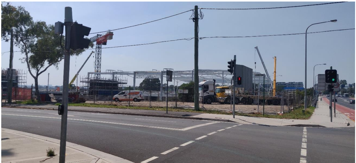
Figure 3: Site viewed from intersection of Victoria Road and Frank Street.
