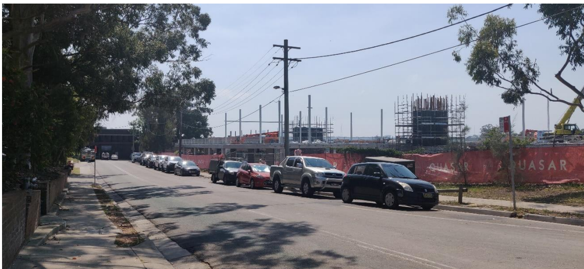
Figure 5: Looking north-east along Frank Street.
