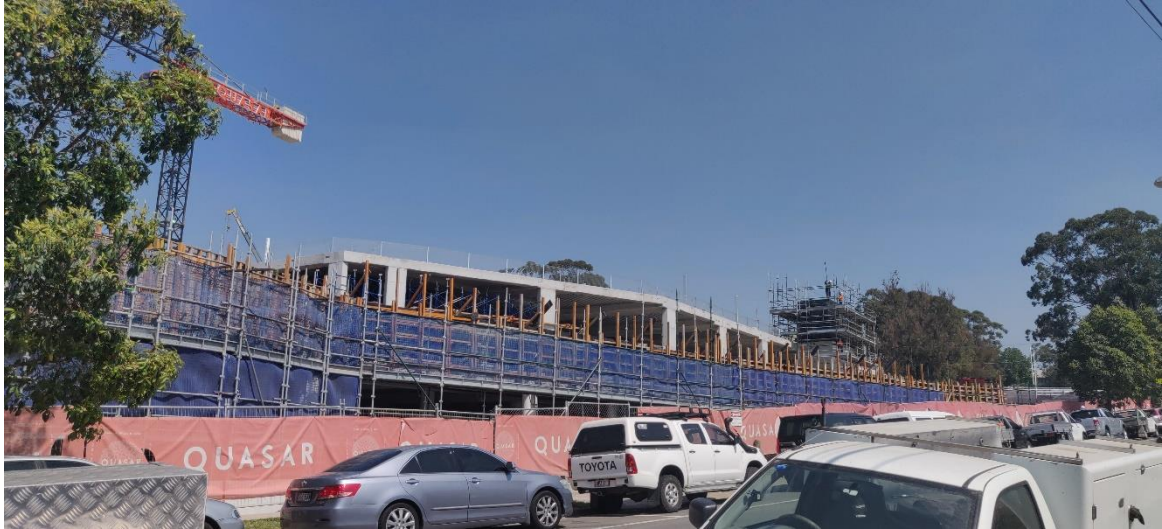
Figure 6: View of Bunnings Warehouse construction works from College Street.
