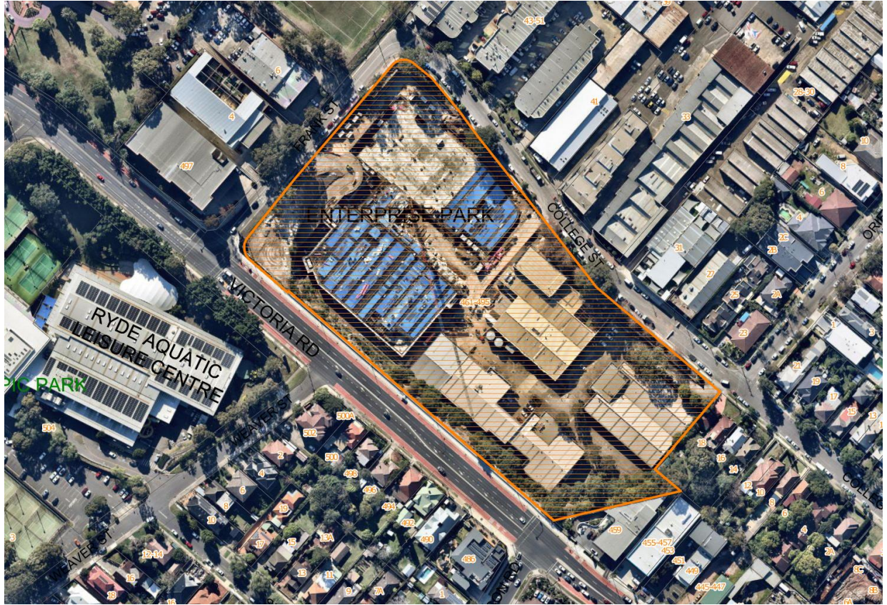
Figure 1: Aerial view of the subject site in its context.
