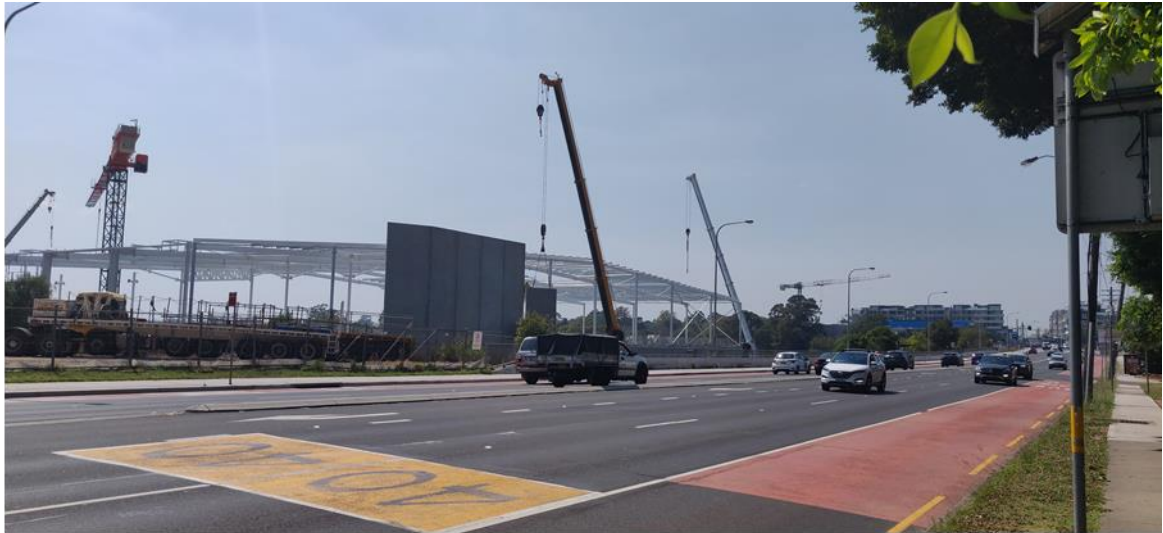
Figure 2: Site viewed from Victoria Road.
