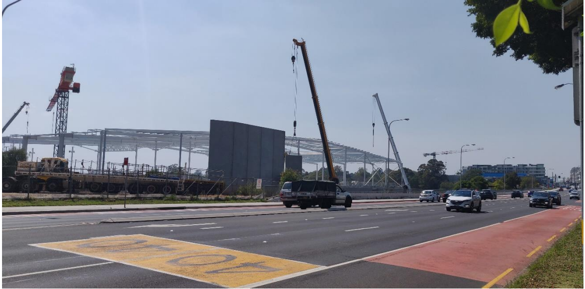
Figure 2: Site viewed from Victoria Road.
