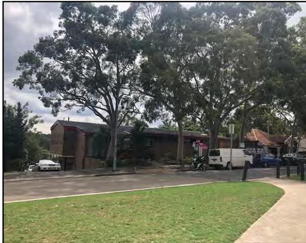
Figure 2: Single storey community centre located at 176 - 178 Blaxland Road.
