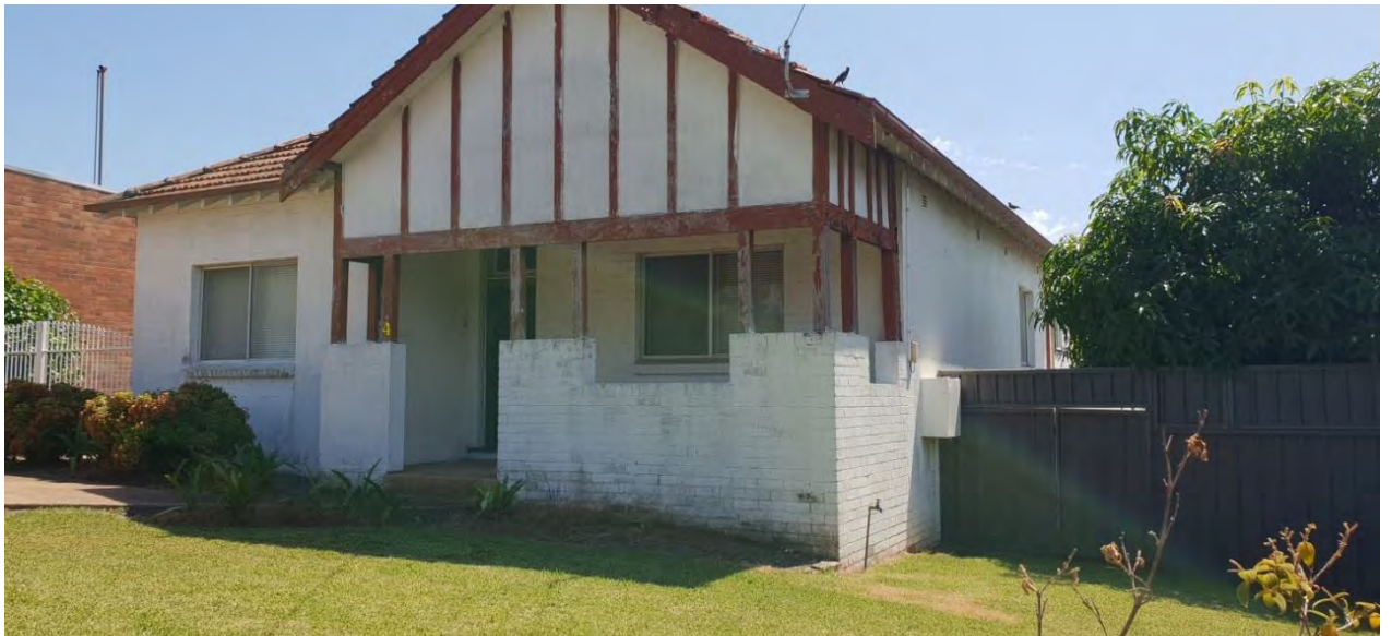
Figure 2: The existing dwelling at the front of the site.
