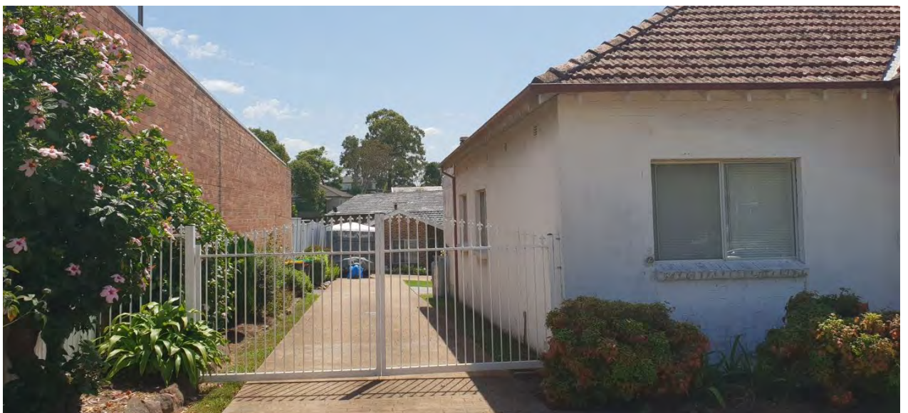
Figure 3: The existing driveway and dwelling at the rear of site.
