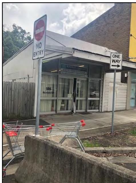
Figure 5: Single storey shop located at 186 Blaxland Road.
