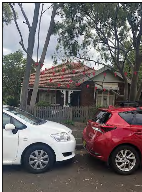
Figure 3: Single storey dwelling located at 182 Blaxland Road.
