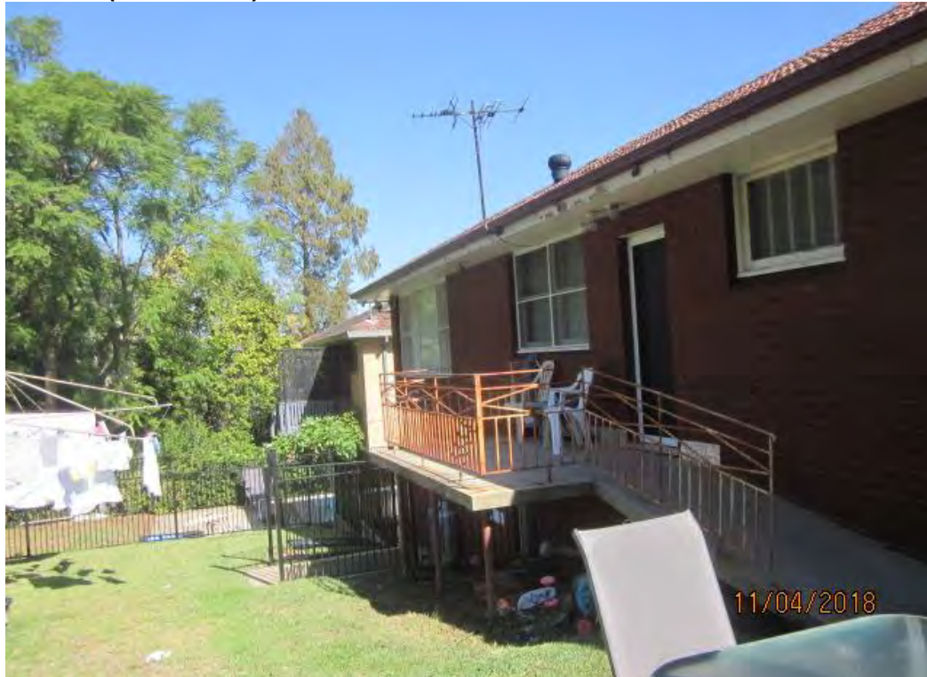
Figure 4: View at rear of existing dwelling.
