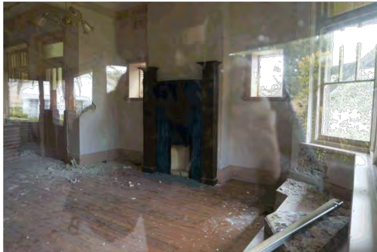
Figure 52: The lounge room and lounge room fireplace
