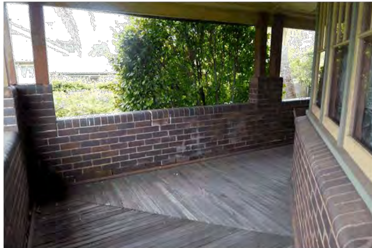
Figure 25: Detail of south-western corner of the return verandah showing brick balustrade, timber posts and timber verandah floor
