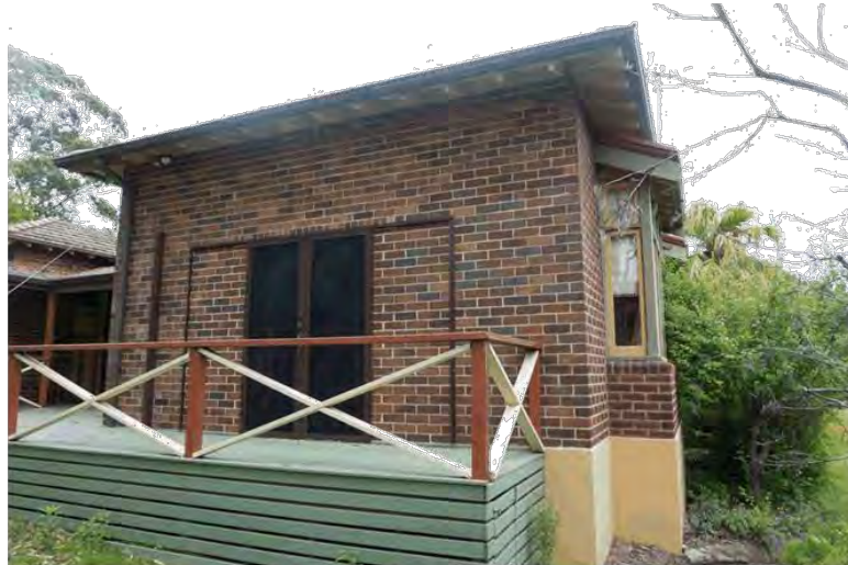
Figure 33: North-west corner of the house
