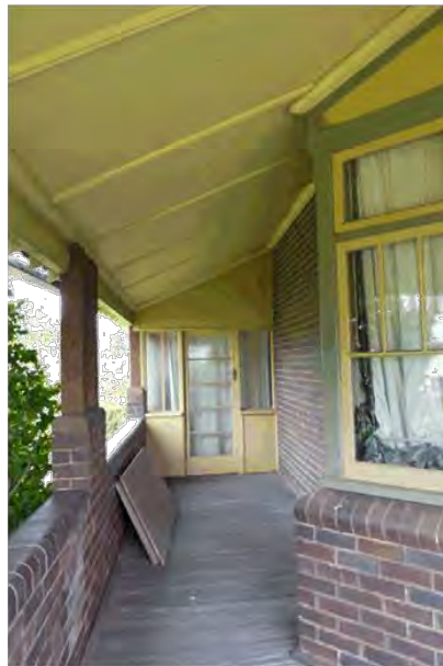
Figure 25: Detail of south-western corner of the return verandah showing brick balustrade, timber posts and timber verandah floor
