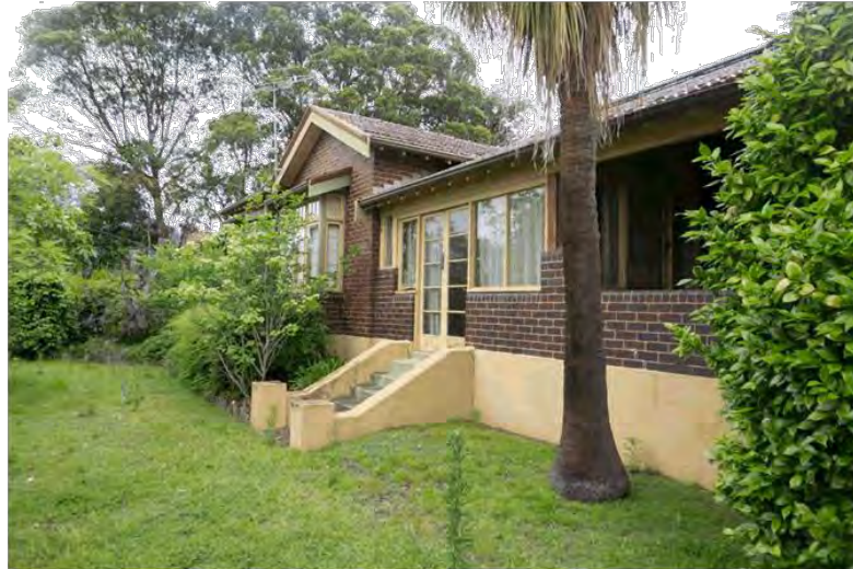
Figure 27: The western elevation of the house, showing the circa 1950s partial verandah enclosure to form a sunroom (centre) with the original western steps onto the verandah remaining.
