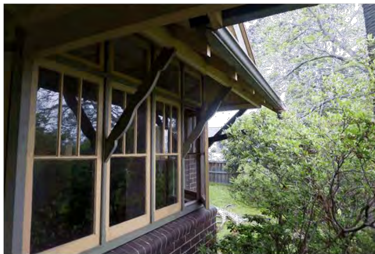
Figure 24: Detail of timber-framed casement windows with fanlights.
