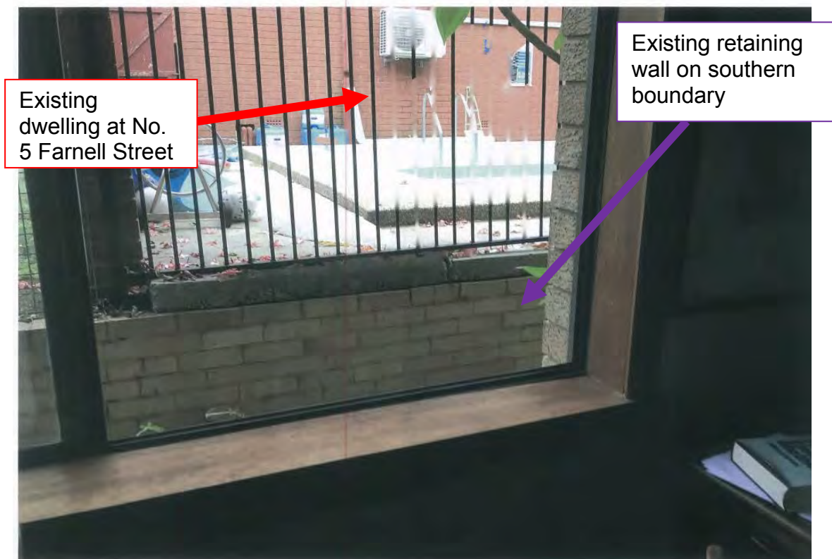
Figure 23: View of existing retaining wall from No. 7 Farnell Street
