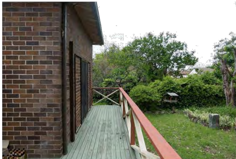
Figure 34: View along the rear (north) elevation looking west with recent decking
