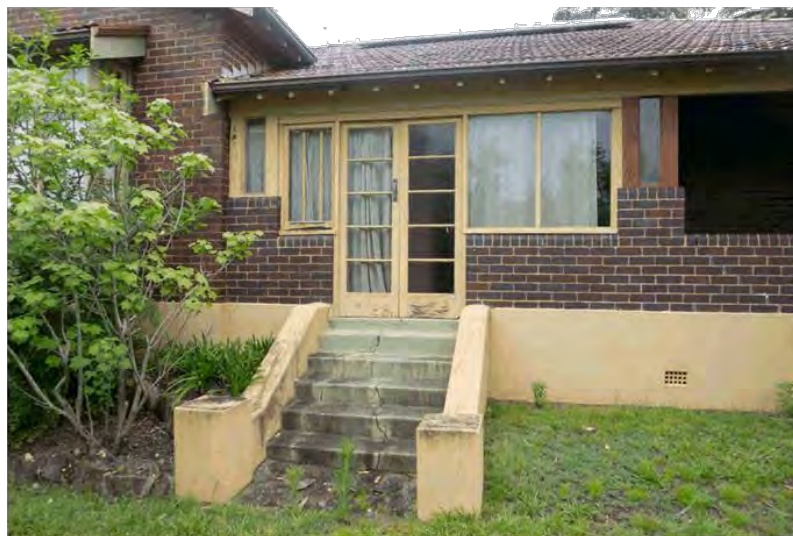
Figure 28: Detail of western verandah circa 1950s sunroom enclosure and original western steps onto verandah.
