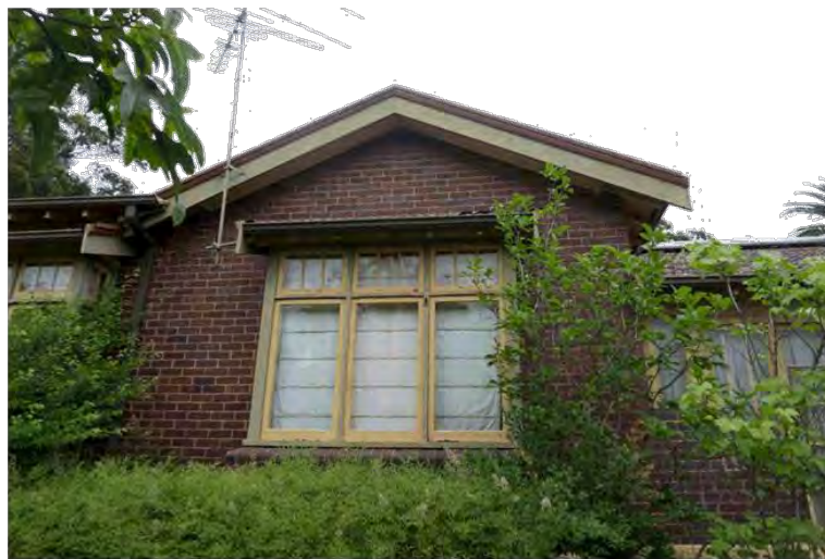
Figure 30: Detail of gable ends, windows and awning on the western elevation of the house.
