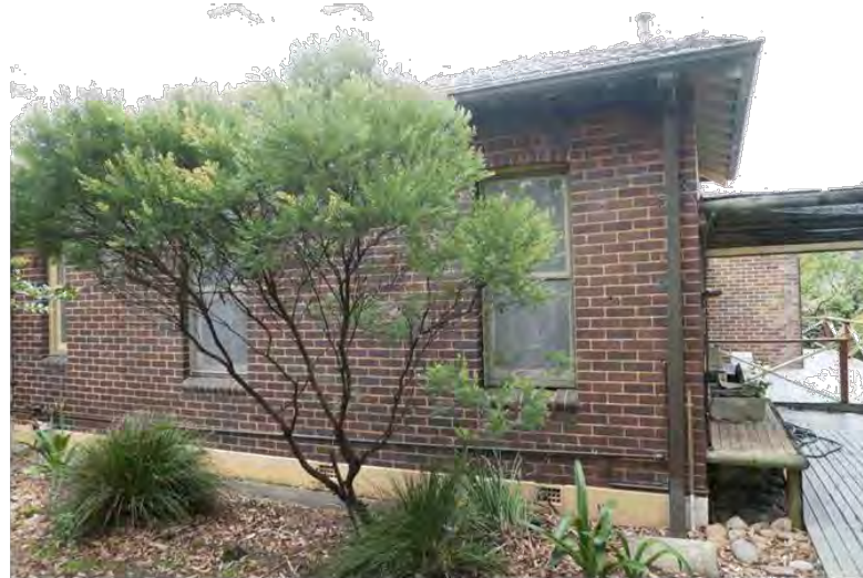
Figure 37: (Left) the north-eastern corner of the house. The two windows shown here are to the kitchen (left) and laundry (right)
