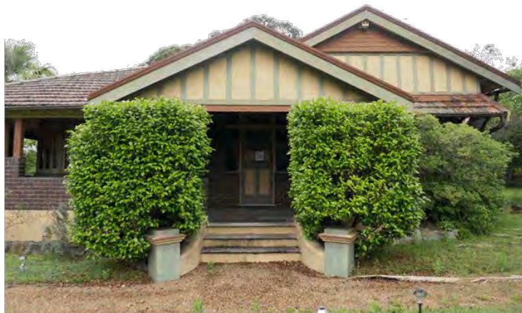
Figure 17: Main front entry to the house from Denistone Road
