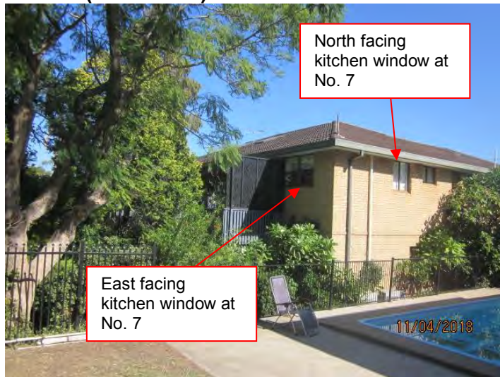
Figure 17: Location of kitchen windows for No. 7 Farnell Street.
