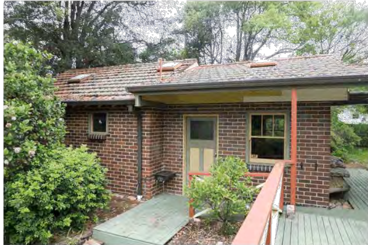
Figure 47: The western elevation of the modern garage (at left) and workshop (at right).
