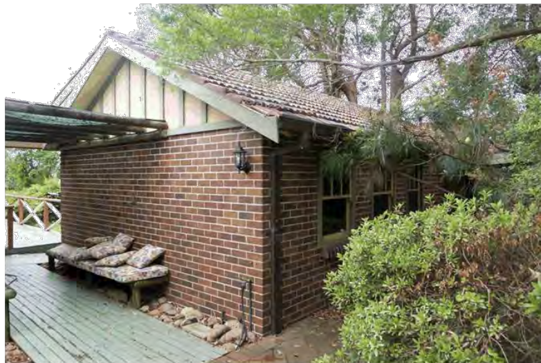
Figure 46: The southern and eastern elevations of the garage/workshop with (at left) the covered area connecting the house to the garage/workshop
