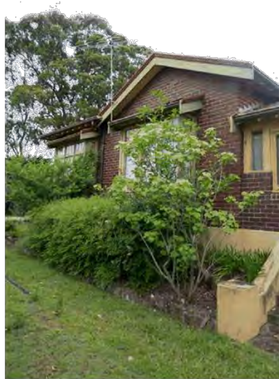
Figure 29: (Left) rear (north) end of the western elevation of the house
