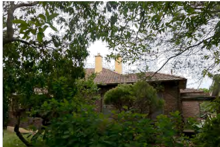
Figure 38: View of the rear of the house from the east, showing the chimneys to the rear of the dining room and to bedroom 3
