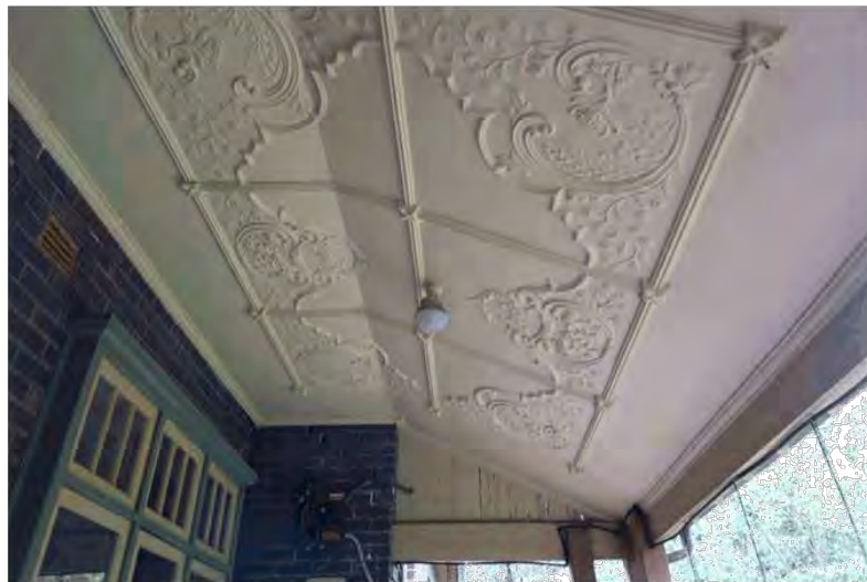
Figure 44: Decorative plaster ceiling to eastern verandah
