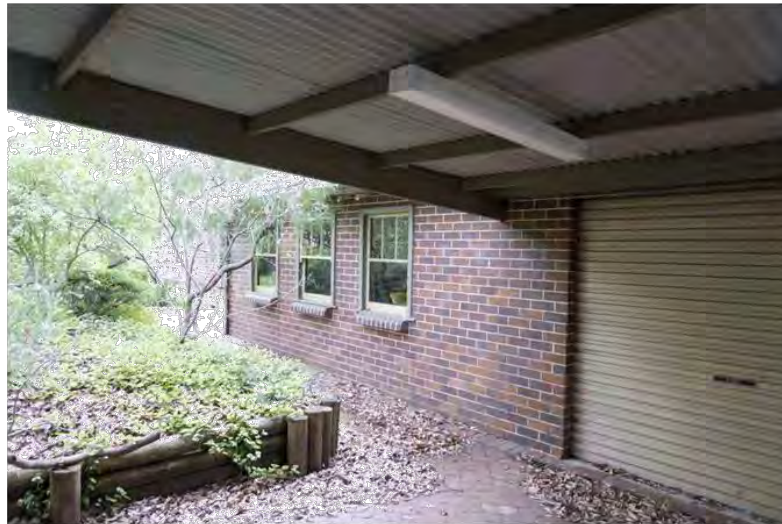
Figure 45: The eastern elevation of the carport and garage/workshop off Florence Avenue
