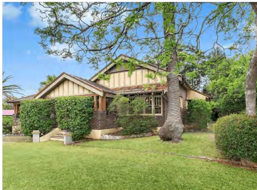
Figure 56: Lanark Brae, 68 Denistone Road, Denistone (corner Florence Avenue)
