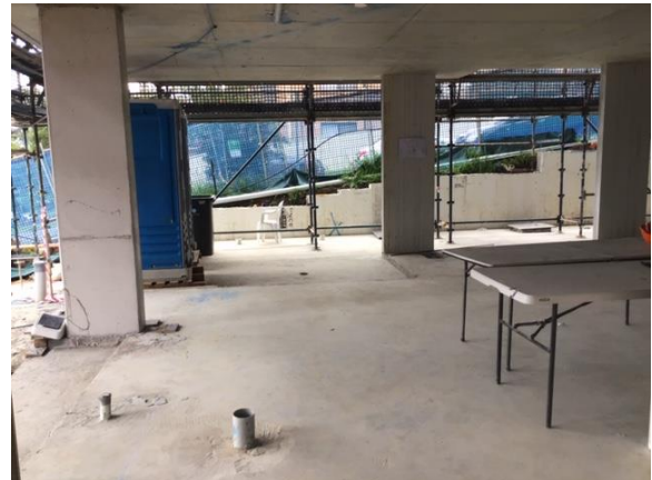
Figure 9 - Unit 01 (View to The Avenue)
