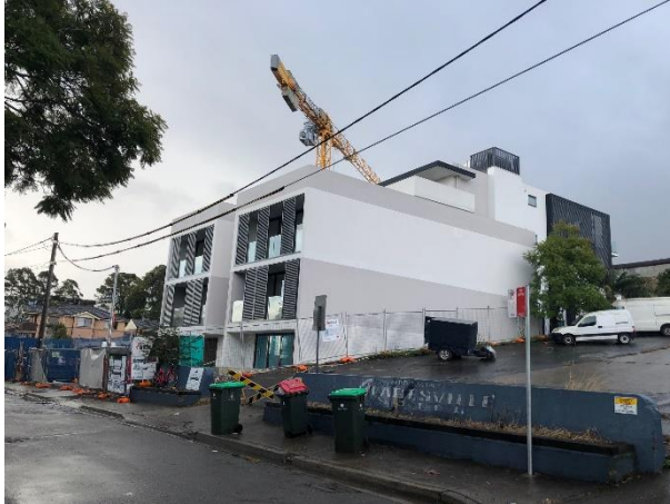
Figure 4 - Photograph of 11 Farm Street.
