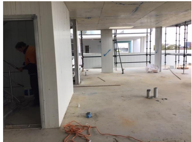
Figure 11 – New Studio Unit 21 (View to the east)
