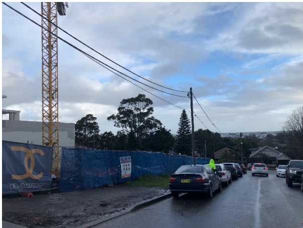
Figure 6 – Pre-construction photograph of the site from The Avenue looking south.
