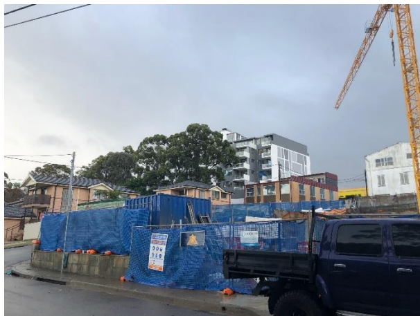
Figure 2 – Pre-construction photograph of the site from Farm Street looking north.
