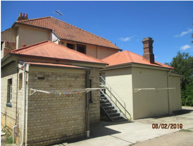
Figure 4. Photo of the south elevation of the existing building.
