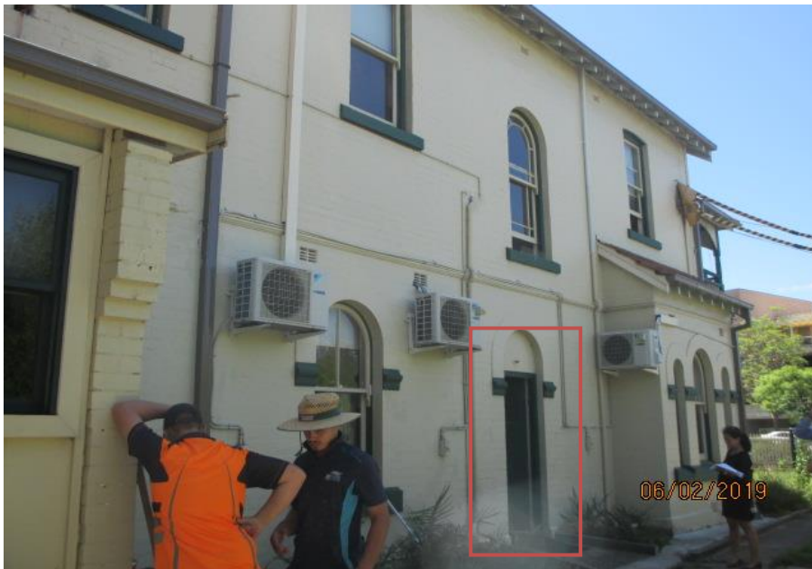
Figure 9. Photograph of existing building identifying primary entrance to access first floor.
