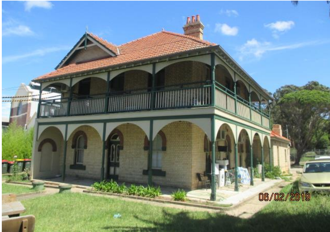
Figure 3. Photo of the heritage listed building on the site, with the Ryde Pumping Station in the background
