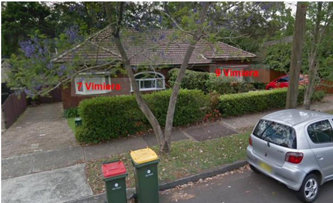
Figure 7: Brick dual occupancy at No. 7-9 Vimiera Rd to the south west
