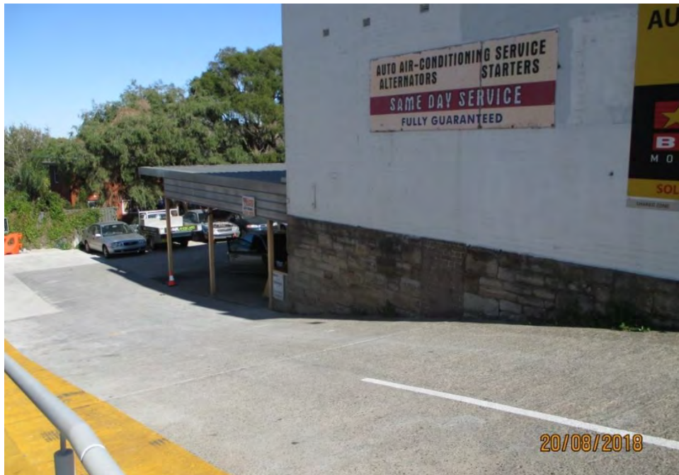
Figure 4: Photograph of building at 744 Victoria Road and existing vehicular access to vehicle workshop at rear of site
