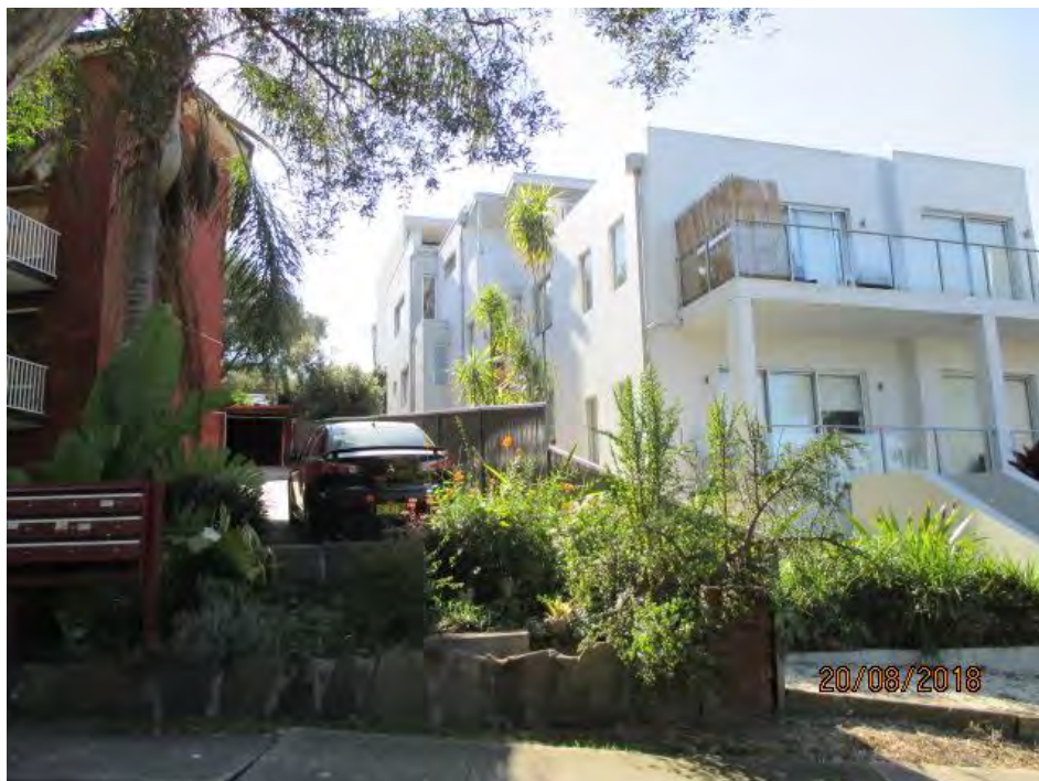
Figure 12: Residential development existing at No. 6 Eagle Street (as viewed from Eagle Street)
