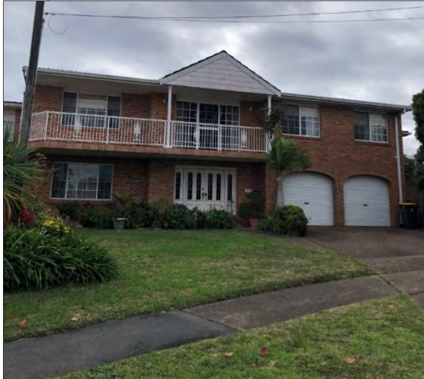
Figure 7: 6 Readford Place, as viewed from Readford Place. Source: CPS Site Inspection, 28 October 2019
