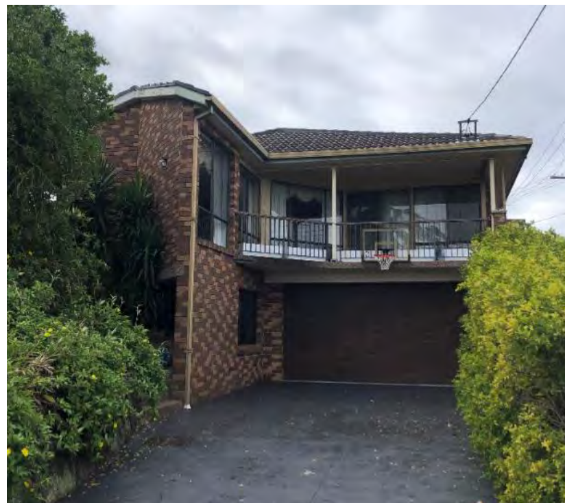
Figure 6: 5 Readford Place, as viewed from Readford Place. Source: CPS Site Inspection, 28 October 2019
