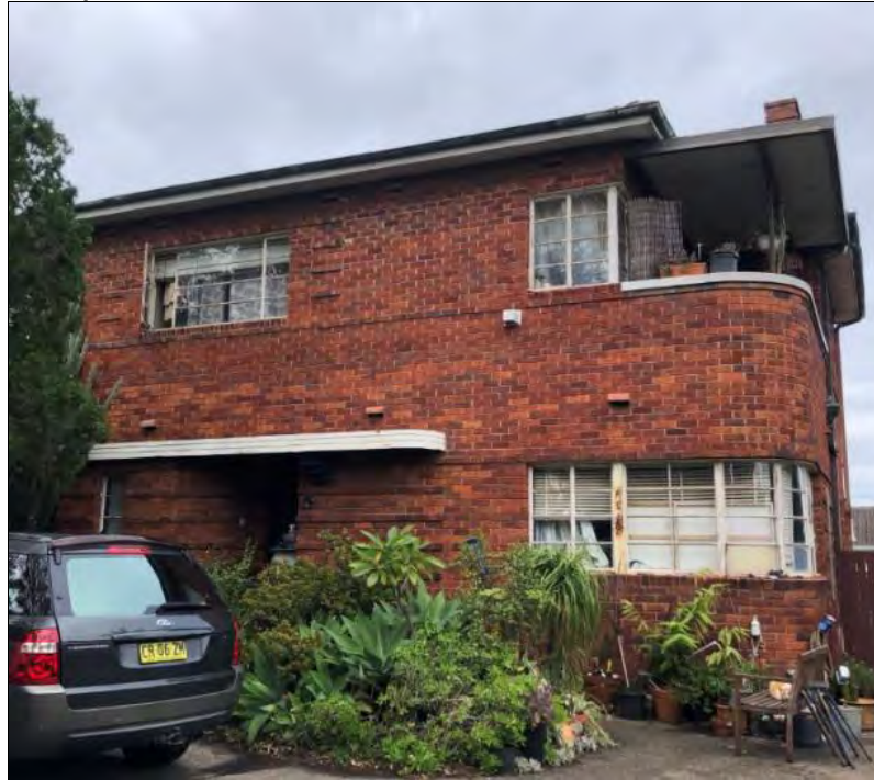
Figure 3: 180 Quarry Road to the northwest of the subject site. Source: CPS Site Inspection, 28 October 2019
