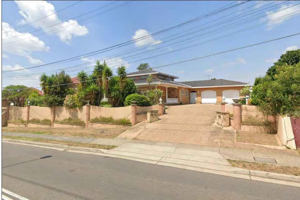
Figure 2: The subject site, as viewed from the northeast within Quarry Road Source: Google, Number 2019
