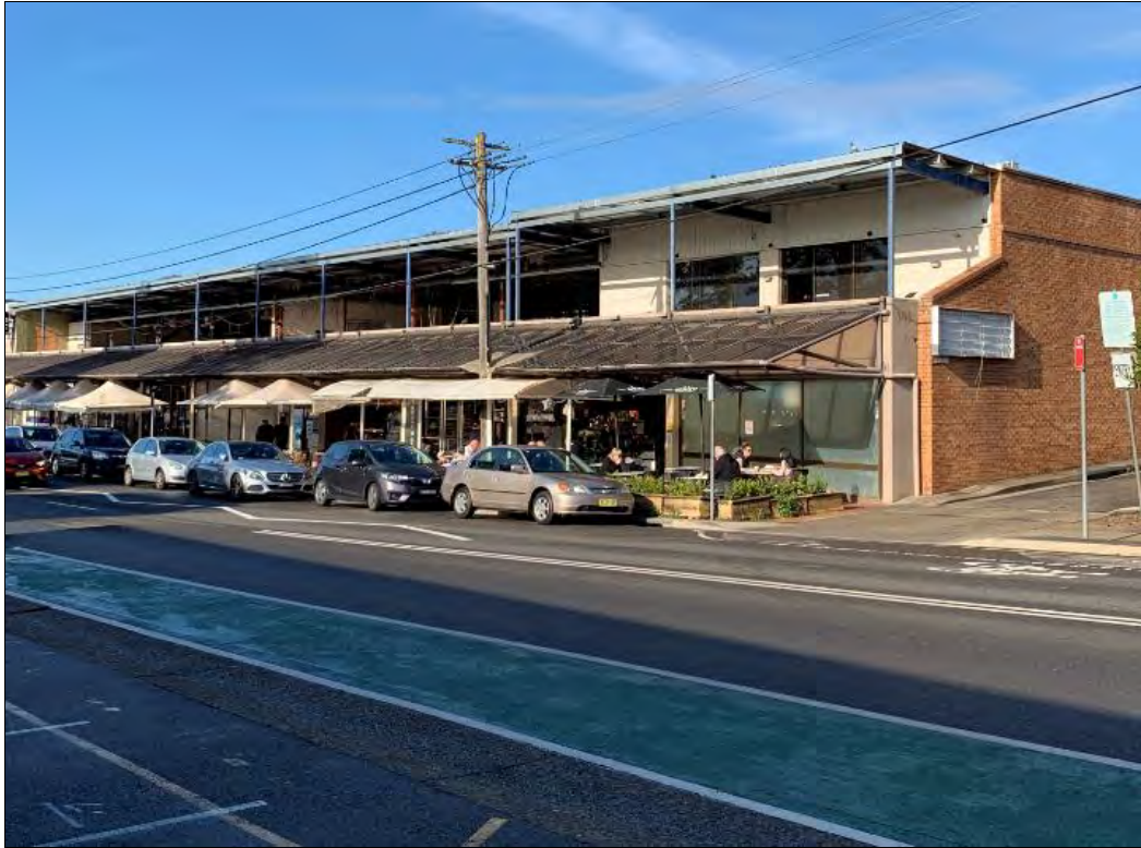
Figure 4 – The subject site, as viewed from the north-eastern side (i.e. opposite side) of Cox's Road. Source: CPS – Site Inspection, 27 June 2019
