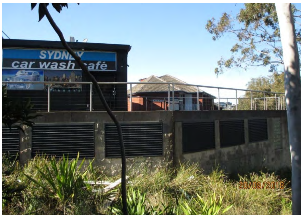
Figure 6: Photograph of existing car wash as viewed from north western corner of site
