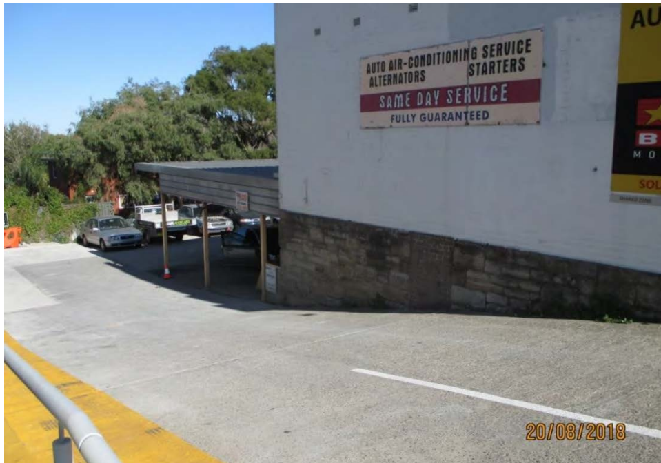
Figure 4: Photograph of building at 744 Victoria Road and existing vehicular access to vehicle workshop at rear of site
