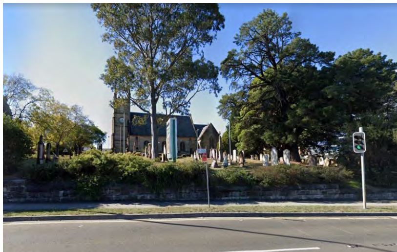
Figure 8: View from Victoria Road of St Anne's Church and cemetery
