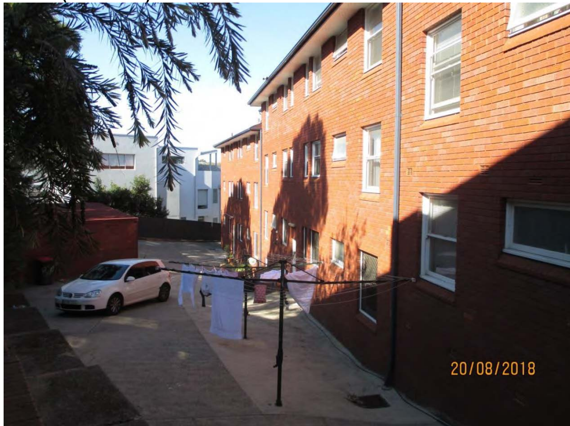
Figure 11: Adjoining RFB located at No. 2 – 4 Eagle Street (rear elevation facing subject site)
