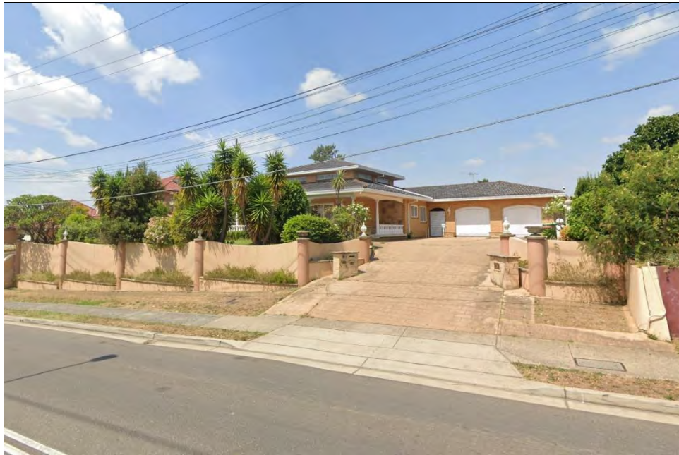
Figure 2: The subject site, as viewed from the northeast within Quarry Road Source: Google, Number 2019
