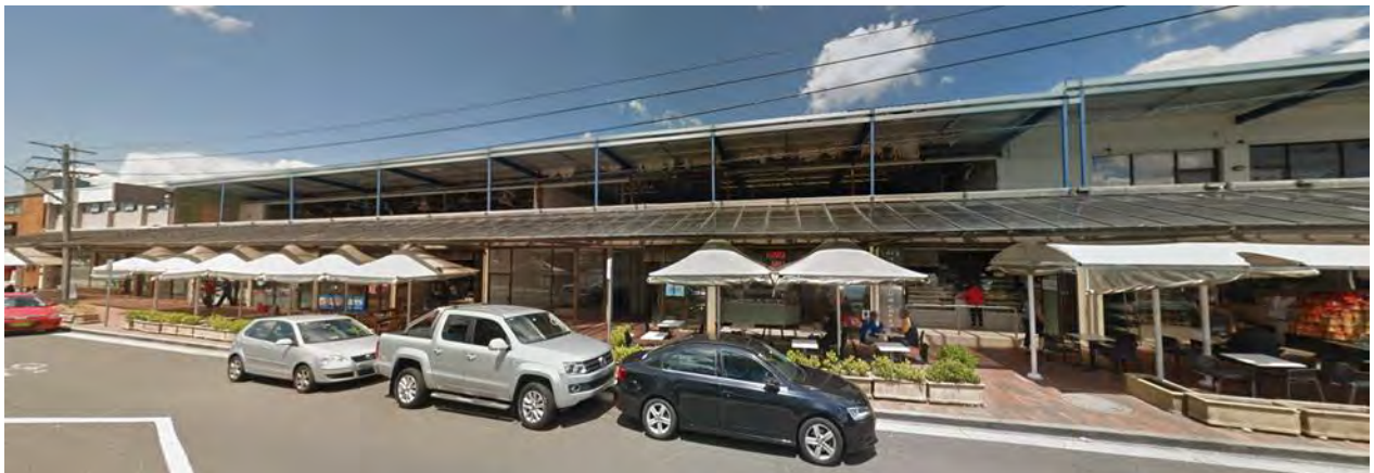
Figure 4 - The existing northern elevation
