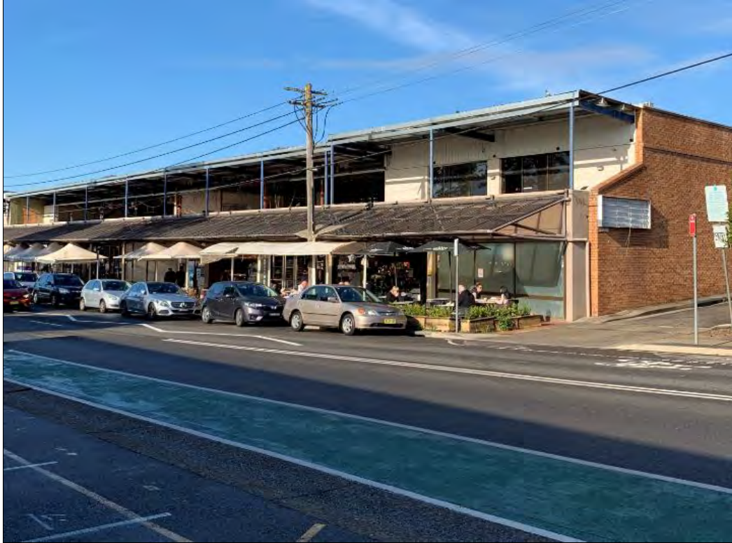
Figure 4 – The subject site, as viewed from the north-eastern side (i.e. opposite side) of Cox's Road. Source: CPS – Site Inspection, 27 June 2019
