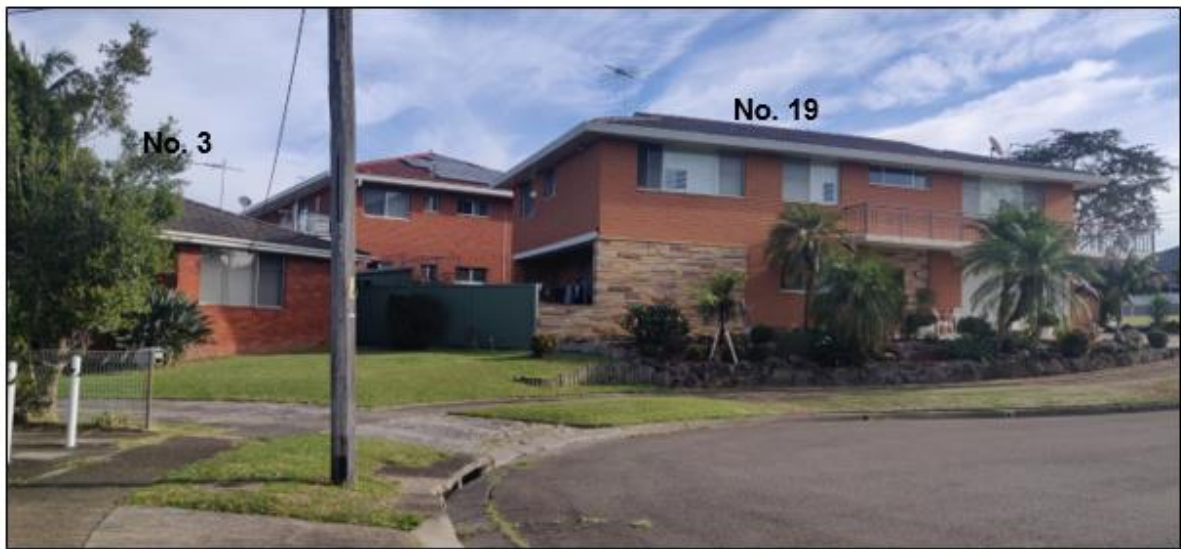
Figure 23: Front setback and landscaping at No. 3 and No. 19 Agincourt Road
