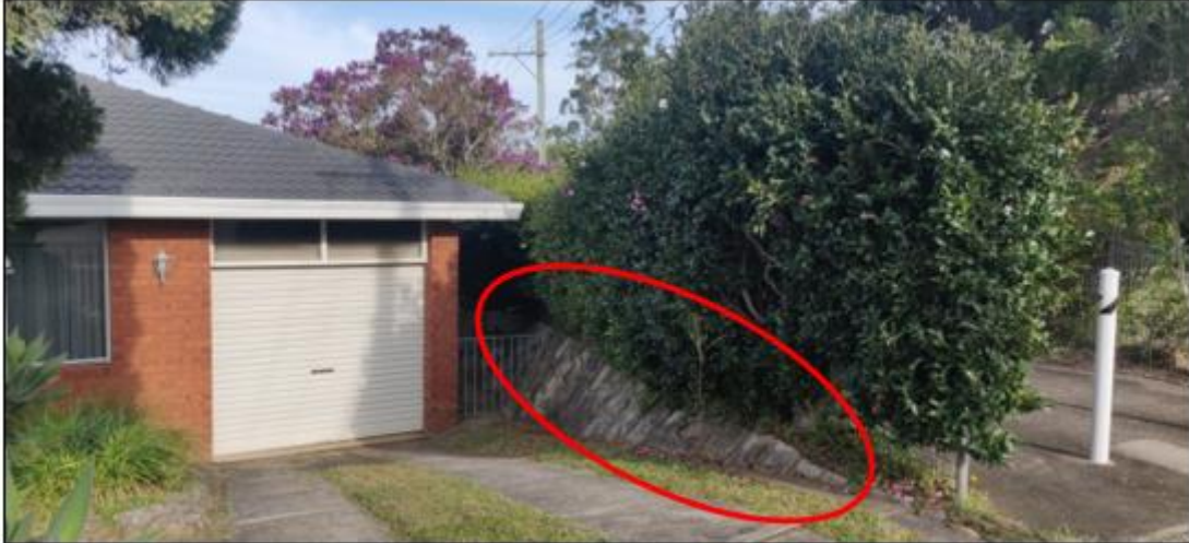
Figure 16: Existing sandstone flagged bank along the southern boundary.
