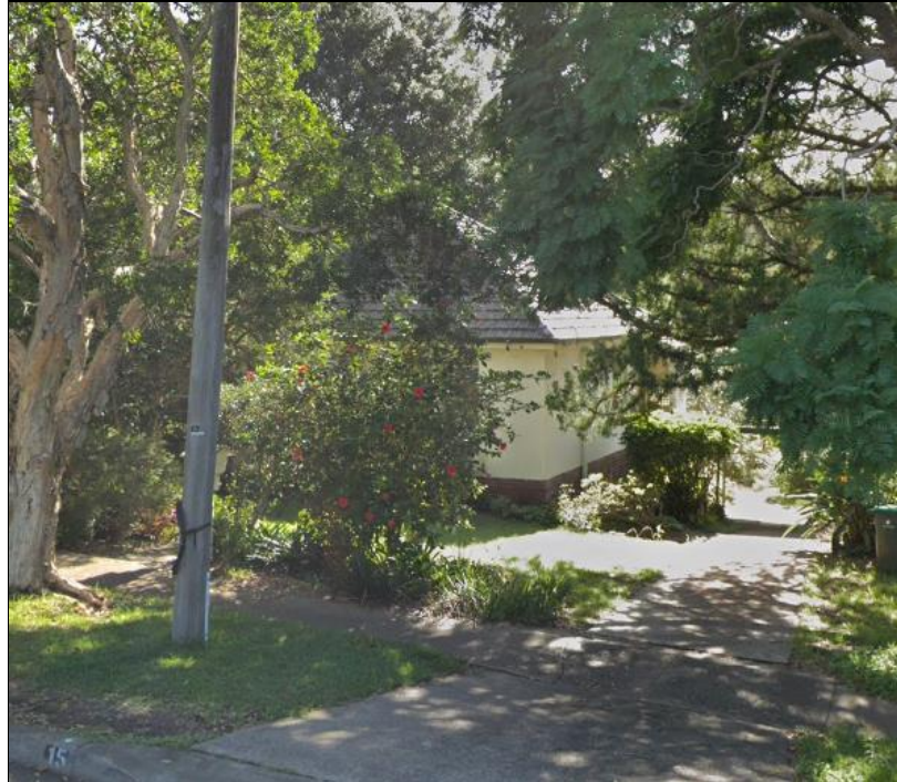
Figure 7: The adjoining part single storey, part two storey dwelling house 15 Miriam Road. Source: Google Maps, March 2019
