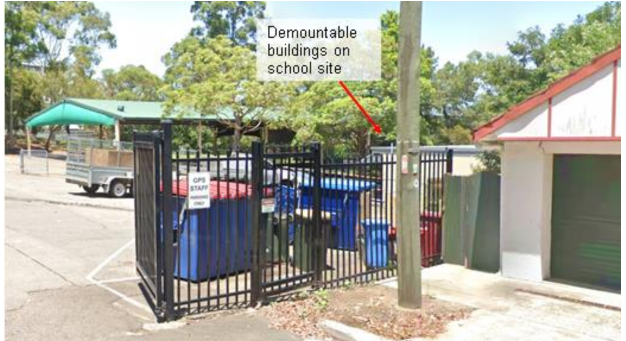
Figure 5: School site directly adjoining subject site (including car park and demountable buildings)
