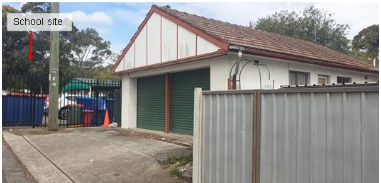
Figure 3: Existing double garage at rear of site
