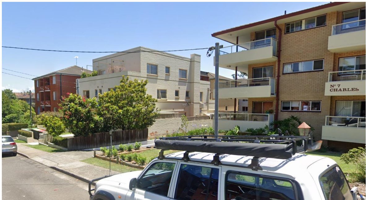
Figure 7: Three storey residential flat buildings on north eastern side of Linsley Street
