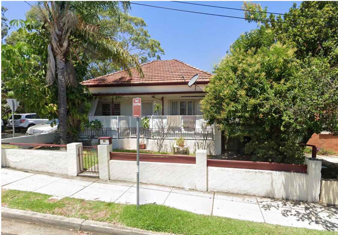
Figure 2: Existing dwelling as viewed from Linsley Street
