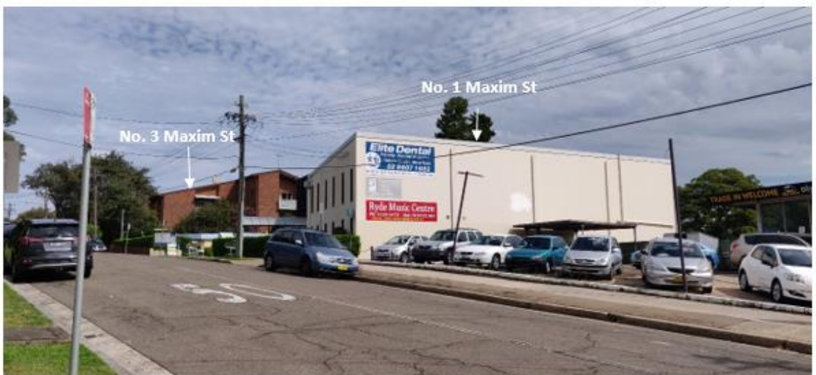
Figure 5: Development immediately south of site on Maxim Street
