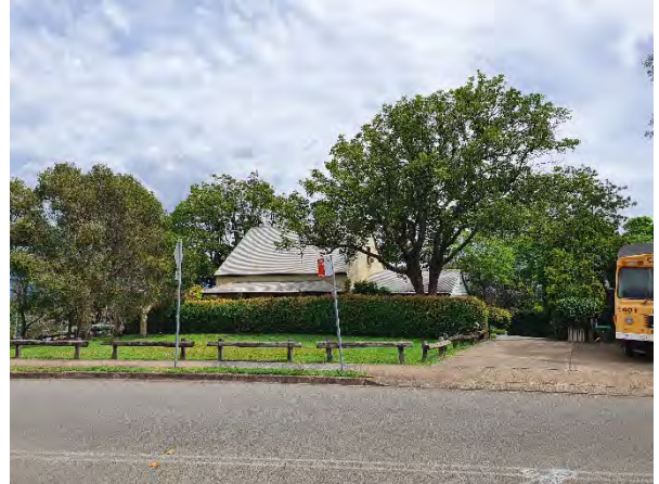
Figure 9. Hatton's Cottage at No. 158 Blaxland Road (west of site).
