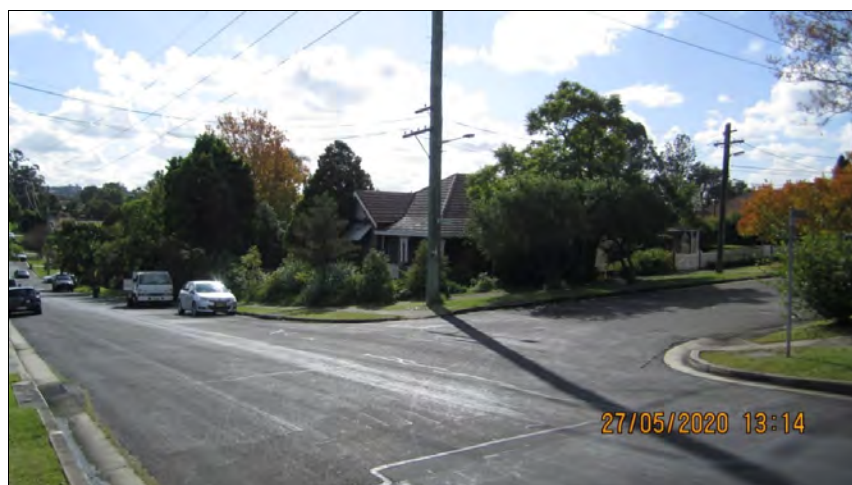
Figure 2 - The site as viewed from Wentworth Road
