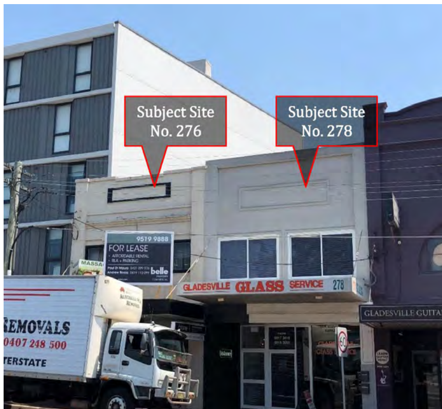
Figure 2: Existing buildings on 276 – 278 Victoria Road.
