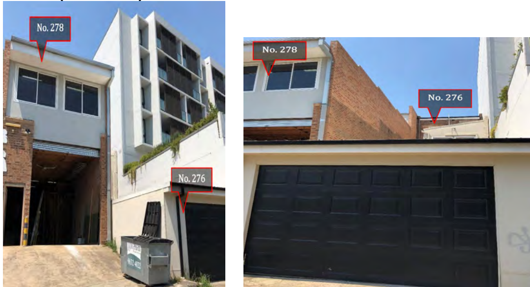
Figure 3: Rear of 276 & 278 Victoria Road – facing Gerard Lane.
