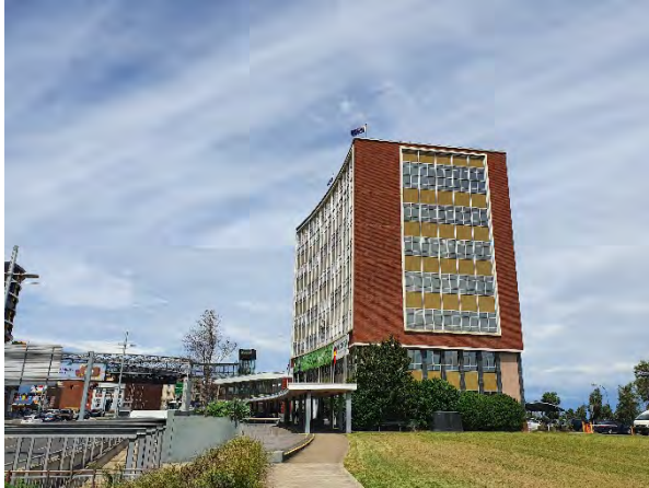
Figure 6. View of the northern side of the existing Civic Centre.
