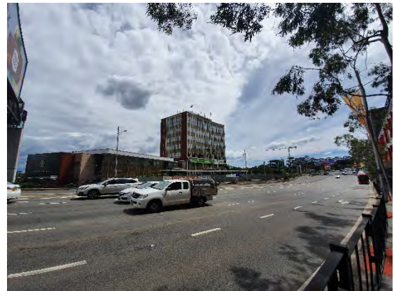
Figure 5. View from the eastern side of Devlin Street.
