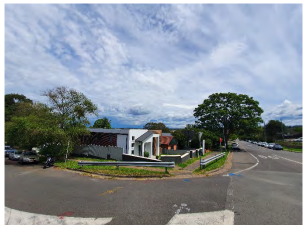
Figure 11. Typical low density residential development off Parkes Street (south west of the site)
