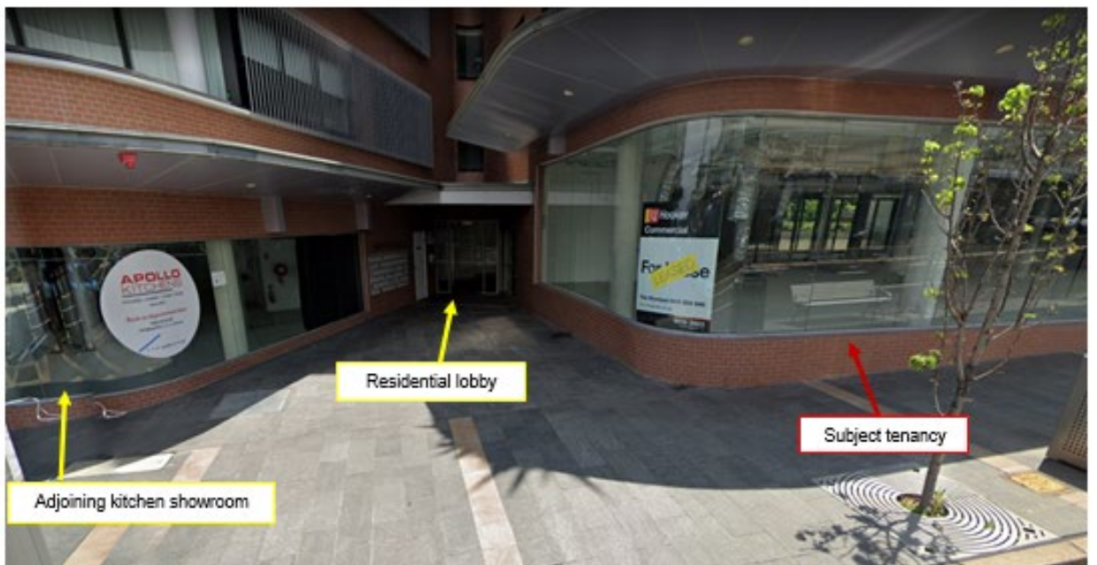
Figure 5: External photograph of subject tenancy and adjoining residential lobby
