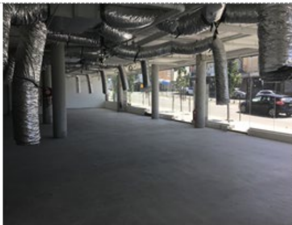
Figure 6: Photograph taken within subject tenancy near entrance (looking toward Victoria Road)
