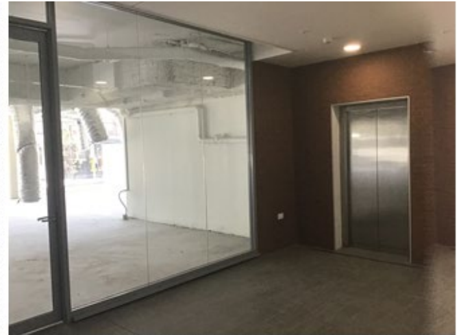
Figure 9: Photograph of lift at rear of tenancy providing access from basement
