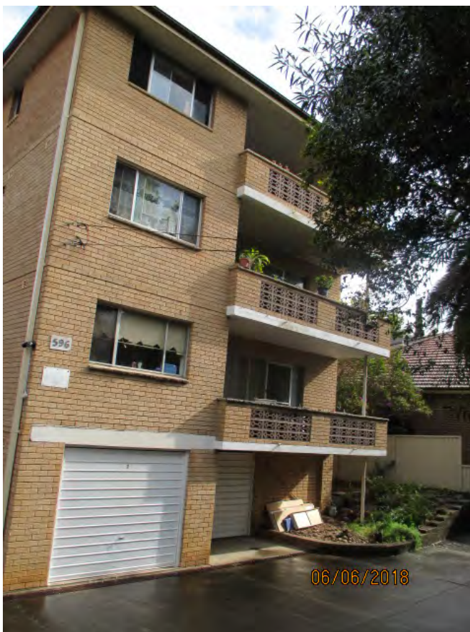
Figure 4: Adjoining southern property - 596 Blaxland Road, 4 storey residential apartment building.
