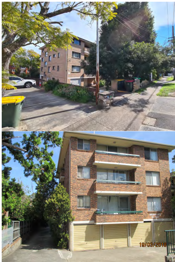
Figure 16: 596 & 600 Blaxland Road with garage under and 3 levels of apartments above. When viewed from the street appears as a 4 storey building.
