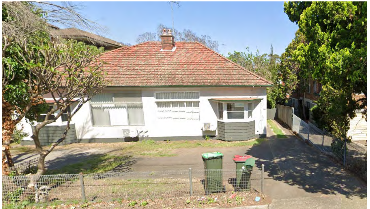
Figure 2: The site as viewed from Blaxland Road – currently contain semi-attached dwellings.
