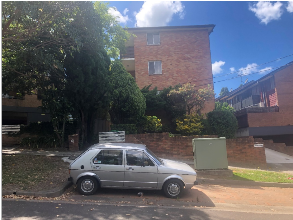
Figure 7 Adjoining property to south west, No. 4 Pearson Street
