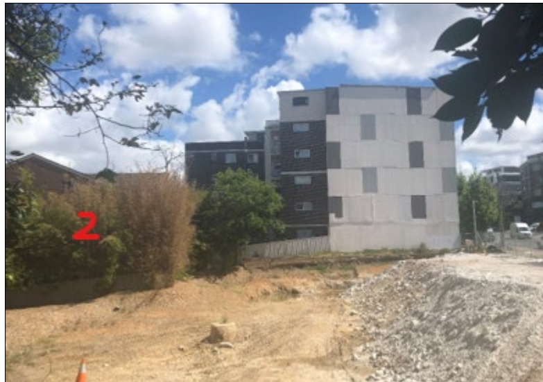
Figure 28 Southern elevation of 120 Victoria Road and 2 Pearson Street behind
