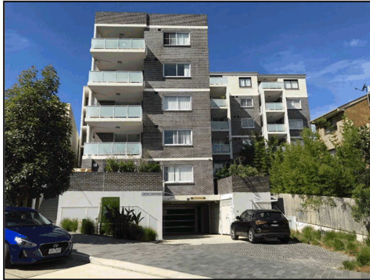
Figure 38: Adjoining property to the north at No. 120 Victoria Road, viewed from Pearson Street
