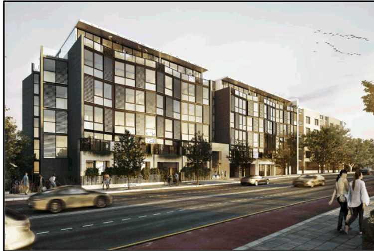
Figure 33: Extract of the photomontage demonstrating the high quality of the proposed development whilst the indiscernible nature of the components which breach the height limit are demonstrated below
