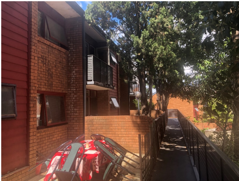
Figure 26 Decking and balconies of 6 Pearson Street presenting to the southern boundary of subject site.
