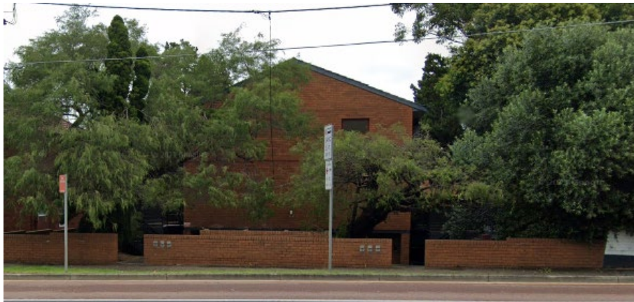
Figure 4 Adjoining site to the south, No. 6 Pearson Street as viewed from Victoria Road
