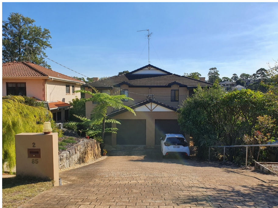
Figure 6 – Adjoining property at 85 and 85B Western Crescent (attached dual occupancy)
