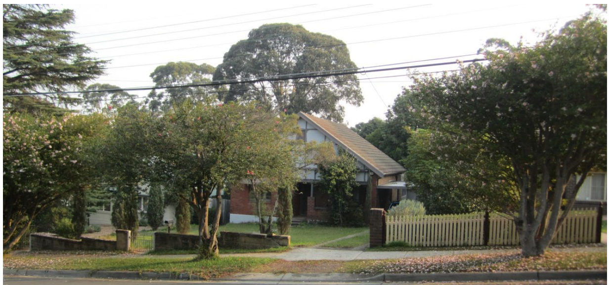
Figure 1: Existing dwelling at 14 Ryedale Road, Denistone
