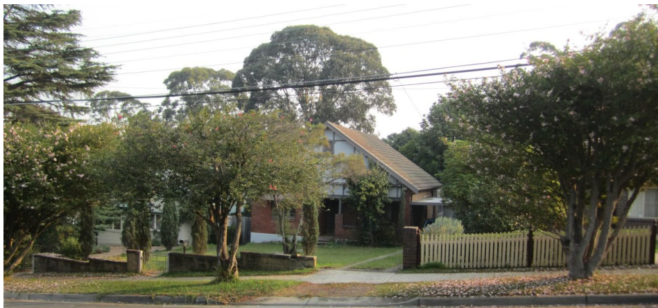
Figure 1: Existing dwelling at 14 Ryedale Road, Denistone
