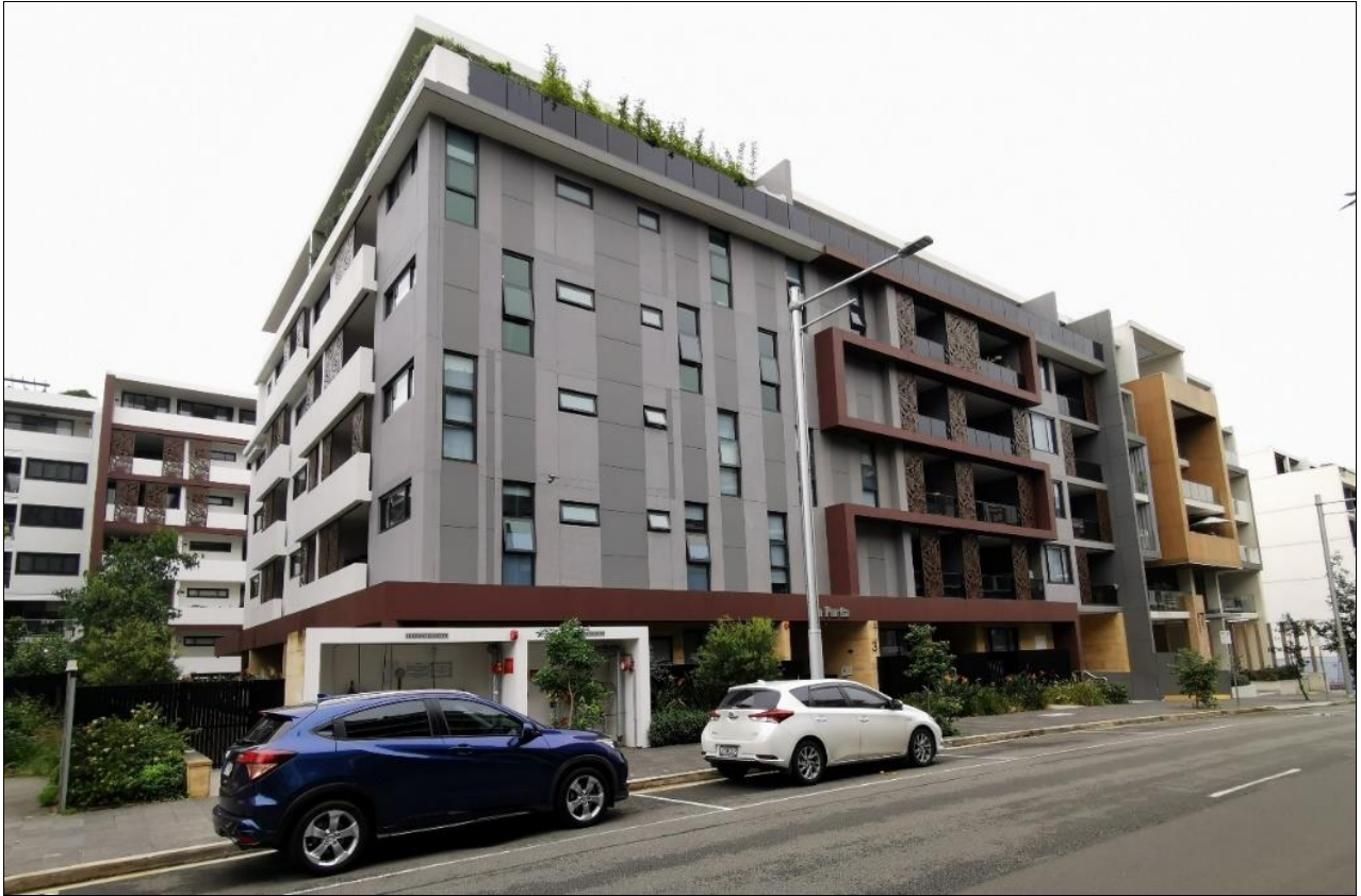
Figure 2: A photo of the subject site as viewed from within the Porter Street road reserve. Source: CPS, 27 April 2022
