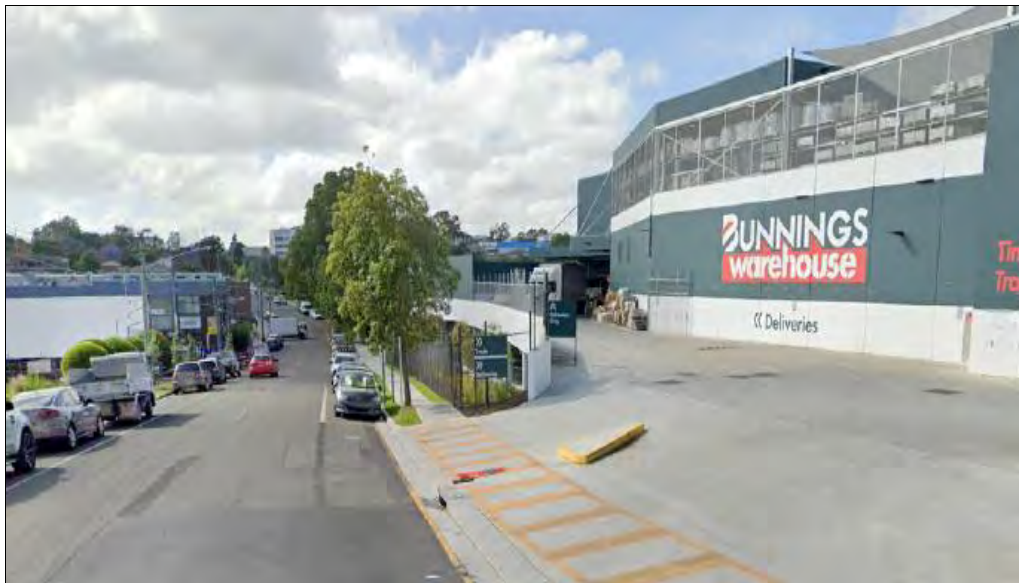
Figure 5 Bunnings building located opposite subject site
