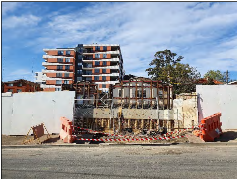
Figure 2 – View of site from Coulter Street depicting excavation and shoring works being undertaken and the rear of the existing Western Crescent facade
