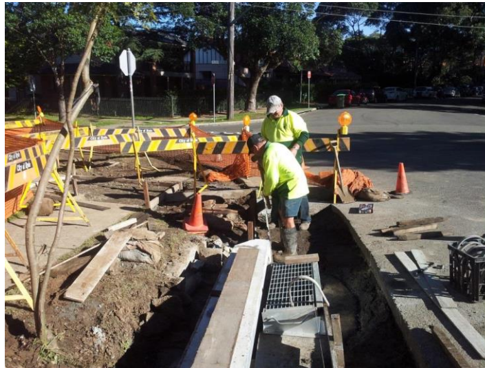
Above: Stormwater asset renewal at Miriam Road, West Ryde. Completed July 2013
