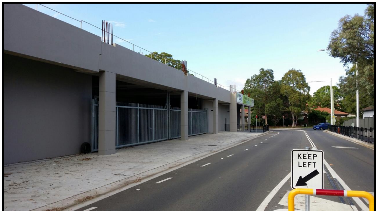
Photograph looking south-west along Betts Street toward Chatham Road. To the left of frame is the partially constructed development at 7-19 Chatham Road where the loading dock is to be located.
