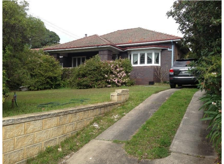
Figure 8: No.492 Blaxland Road. Single Storey Dwelling House – Subject Site.
