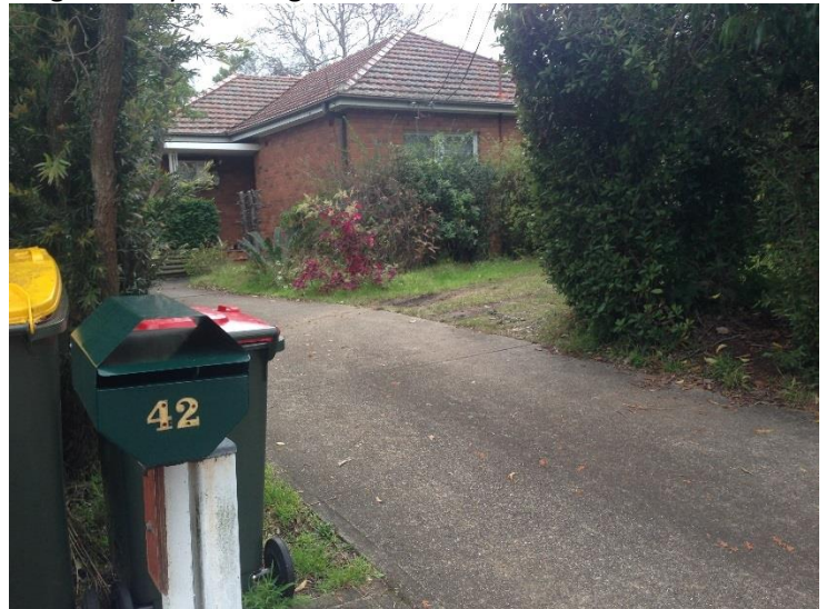
Figure 34: No.42 Denistone Road. Single Storey Dwelling House.
