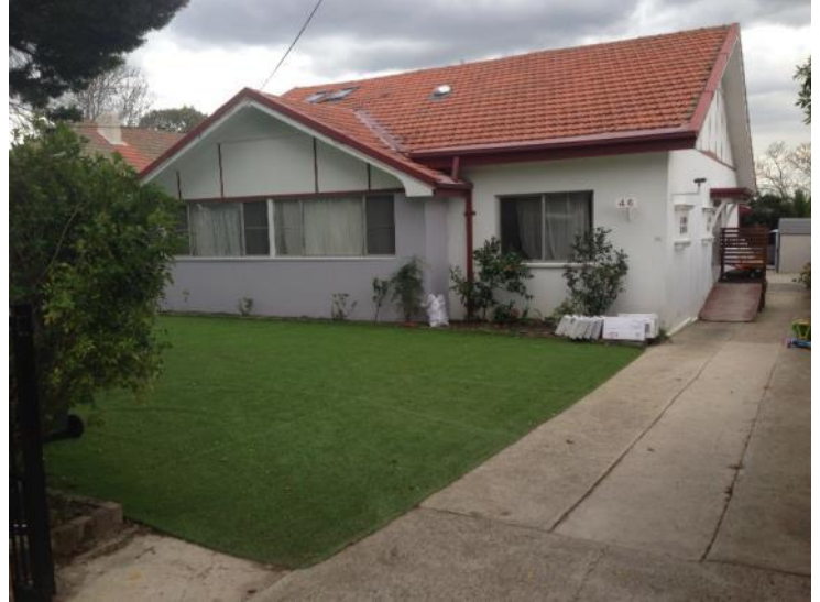
Figure 36: No.46 Denistone Road. Two Storey Dwelling House – Presents to Denistone Road as single storey.
