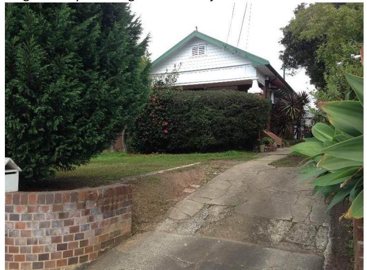
Figure 10: No.488 Blaxland Road. Single Storey Dwelling House.
