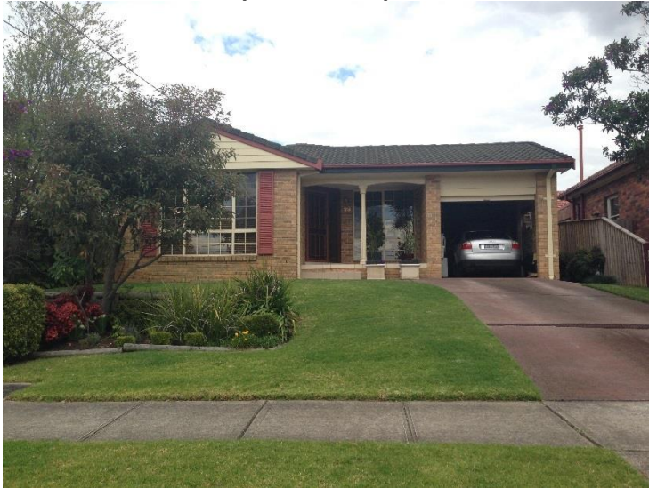
Figure 19: No.28 Hollis Avenue. Single Storey Dwelling House.
