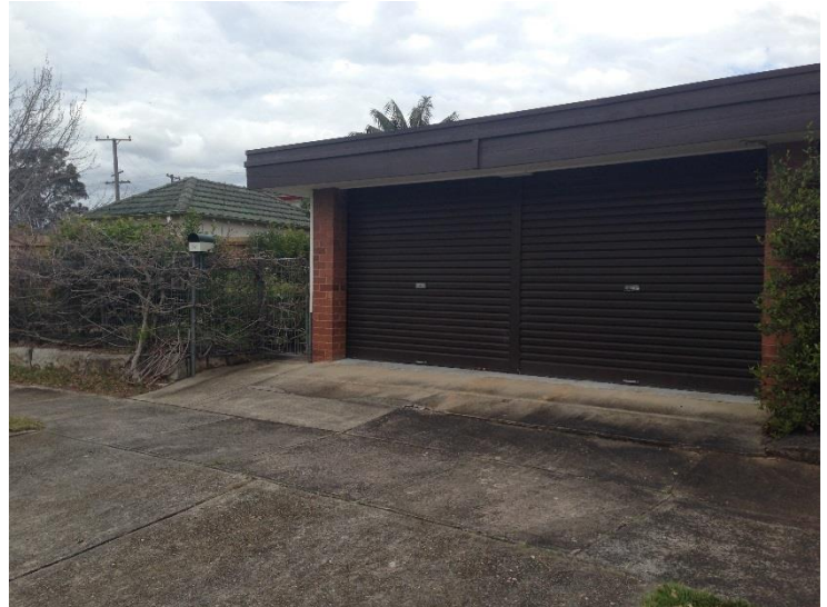
Figure 22: No.34 Hollis Avenue. Single Storey Dwelling House.
