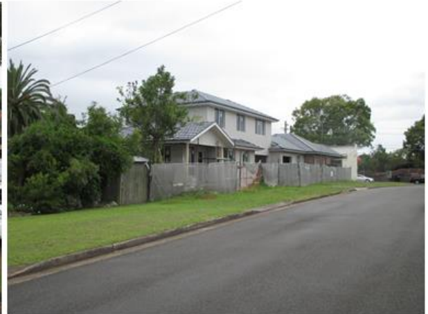
No. 69 Adelaide Street (corner of Deakin and Adelaide Street) (above)
