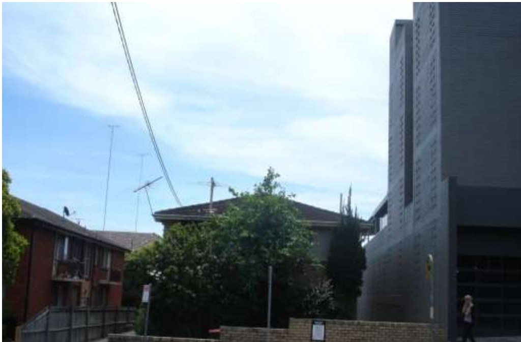
Photograph 1 – Existing Residential Flat Building at 9 Jordan Street in the centre and the western wall of the building at 1-7 Jordan Street on the right of the photo.
