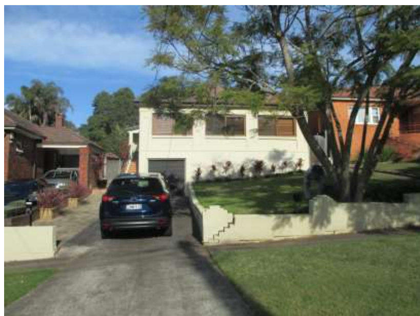
View of subject site from Buena Vista Ave.
