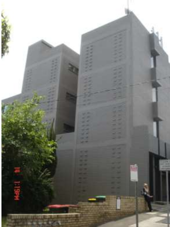
Photograph 2 – Western wall (and light well) of the building at 1-7 Jordan Street.
