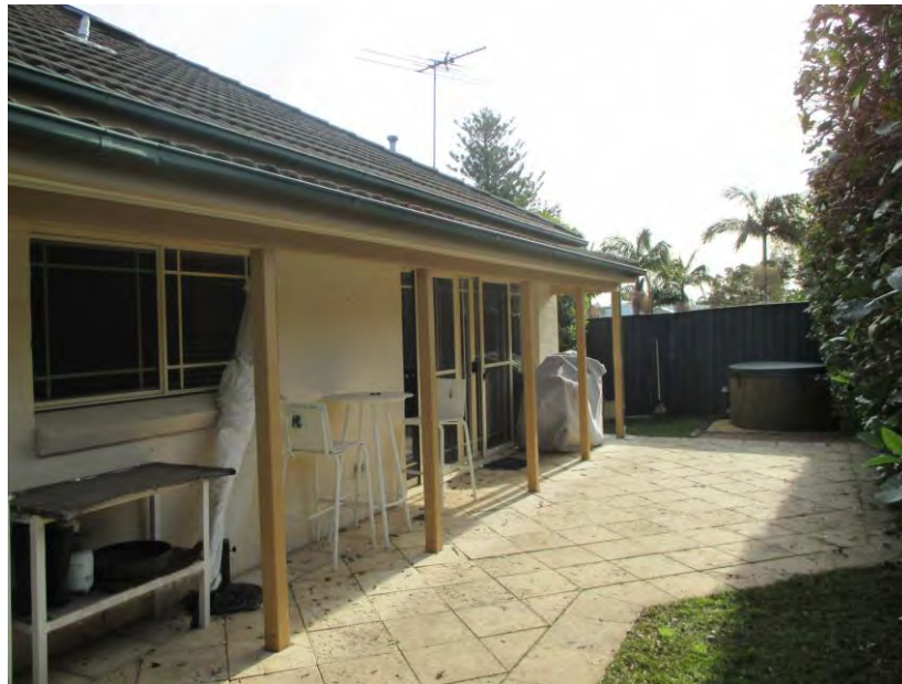
View of paved outdoor terrace
