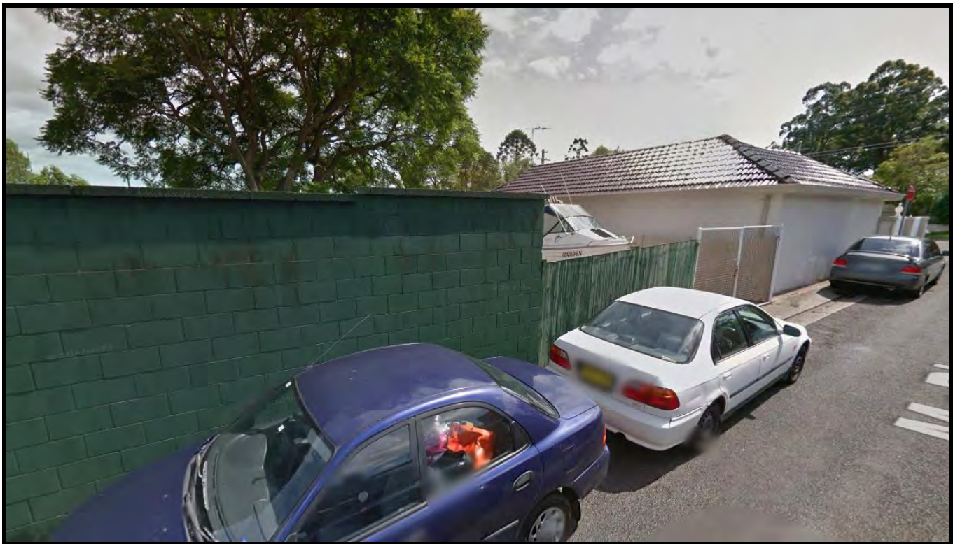
Figure 7 – Image showing zero setbacks to Macpherson Lane opposite the subject site. Numerous buildings with zero setbacks are identified along Macpherson Lane. As such the proposed zero setback is not considered uncharacteristic of the laneway. Source: Macpherson www.google.com
