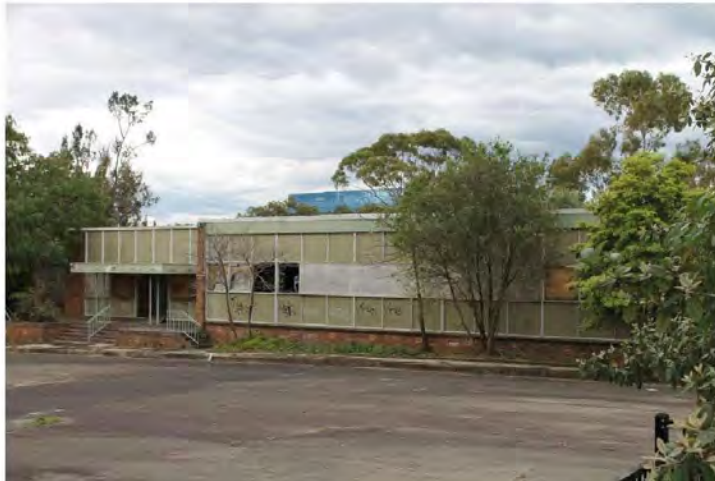
Figure 3 – Existing building at the site
