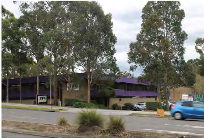
Figure 10 – 'TPG' building to the west of the site
