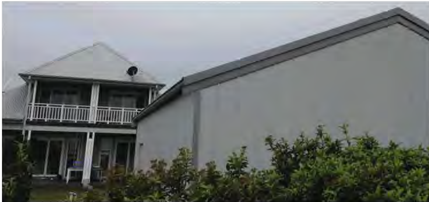
Figure 2: Existing shed (to the right) to the rear of the dual occupancy (to the left) as seen from over the fence from 7A Searle Street
