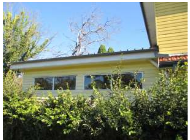
2. External - Living Room windows No.5
