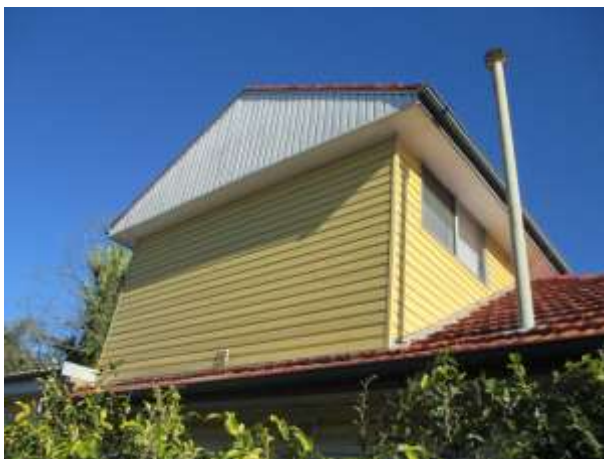
1. External - First floor No.5 facing No.7
