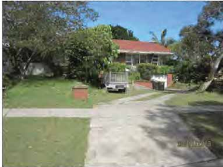
View of subject site from Winbourne Street.
