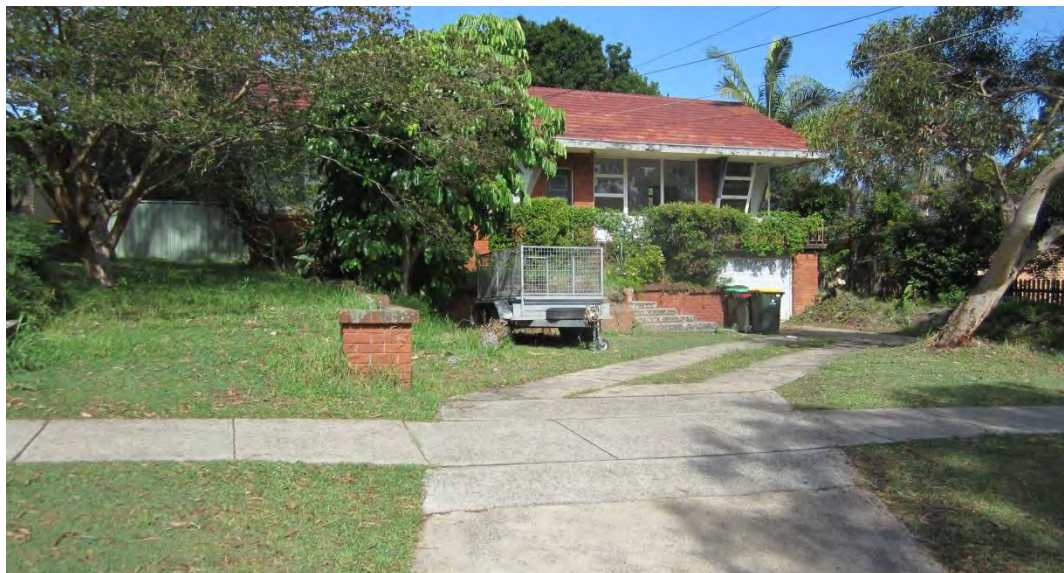
View of subject site from Winbourne Street.
