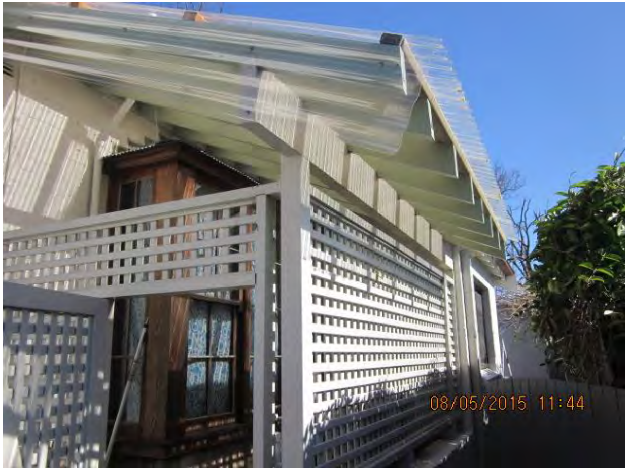
Figure 6: 10 Reserve Street (existing north facing windows).
