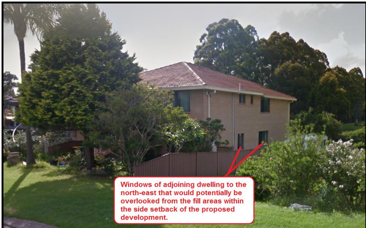
Figure 5 –This diagram shows the adjoining dwelling house to the north-east of the subject site at 91 Culloden Road which is directly opposite the fill proposed at the shared zone for the disabled car parking space in the side setback. Noted is the adjoining windows which may be overlooked from persons in the shared zone and accessing the side setback area of the subject site. As such a privacy screen is recommended adjacent to the elevated shared parking zone to prevent overlooking and subsequent loss of privacy.
