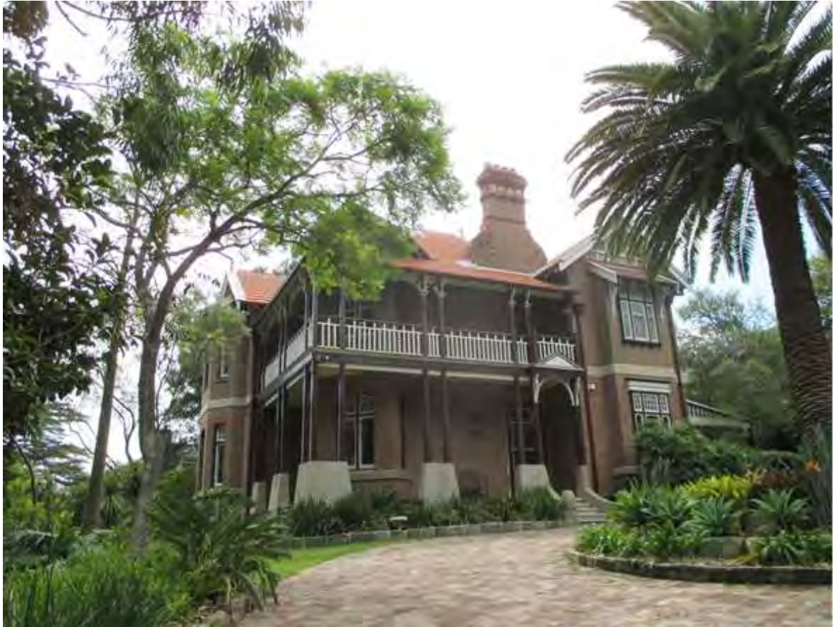
View of subject site from Pennant Avenue.
