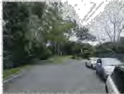
Figure 3.1 View southward 37 Pennant Avenue, showing the split level road arrangement. Source: OCP Architects 2014
