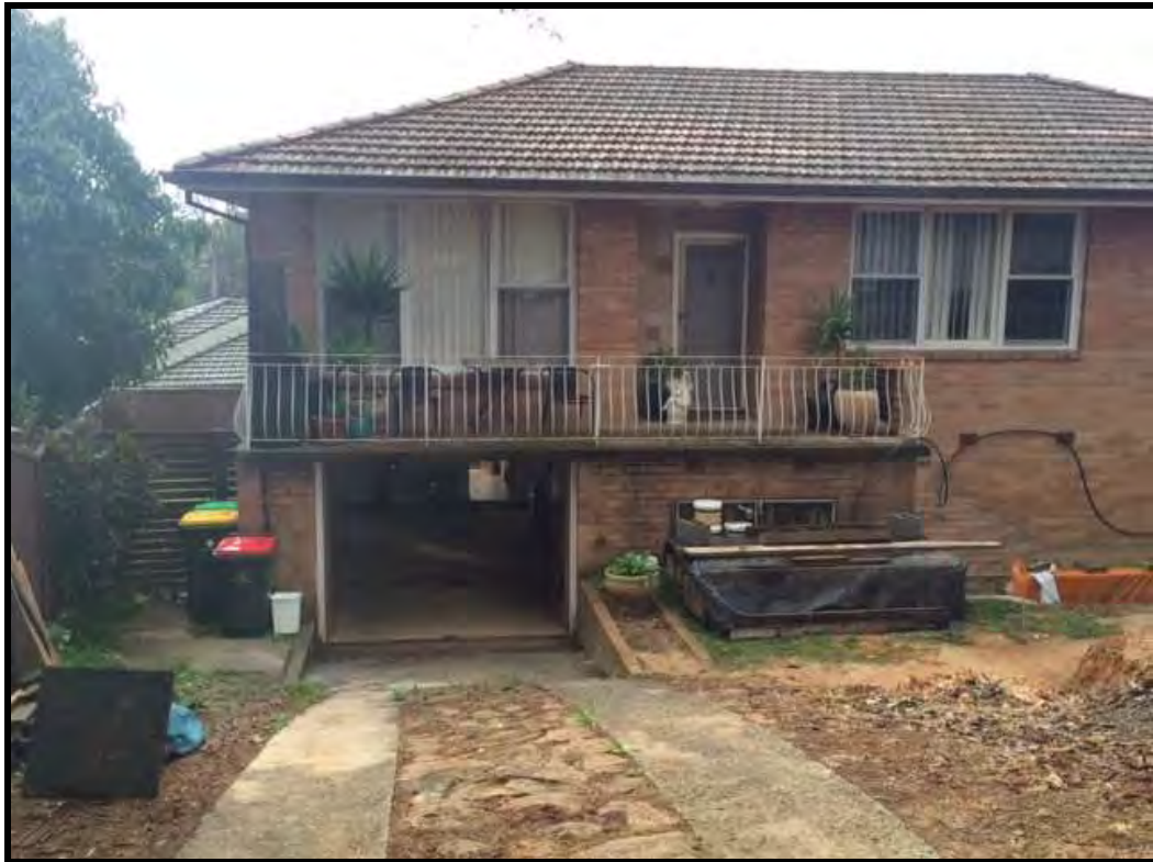
Figure 2 – View of subject site from the Conrad Street frontage. Noted in this image is the existing garage on the ground floor of the dwelling. Also noted is the existing front balcony which demonstrates a prevailing level of overlooking inherent to subject site and adjoining property at No.36 Conrad Street. Source: CPS photograph
