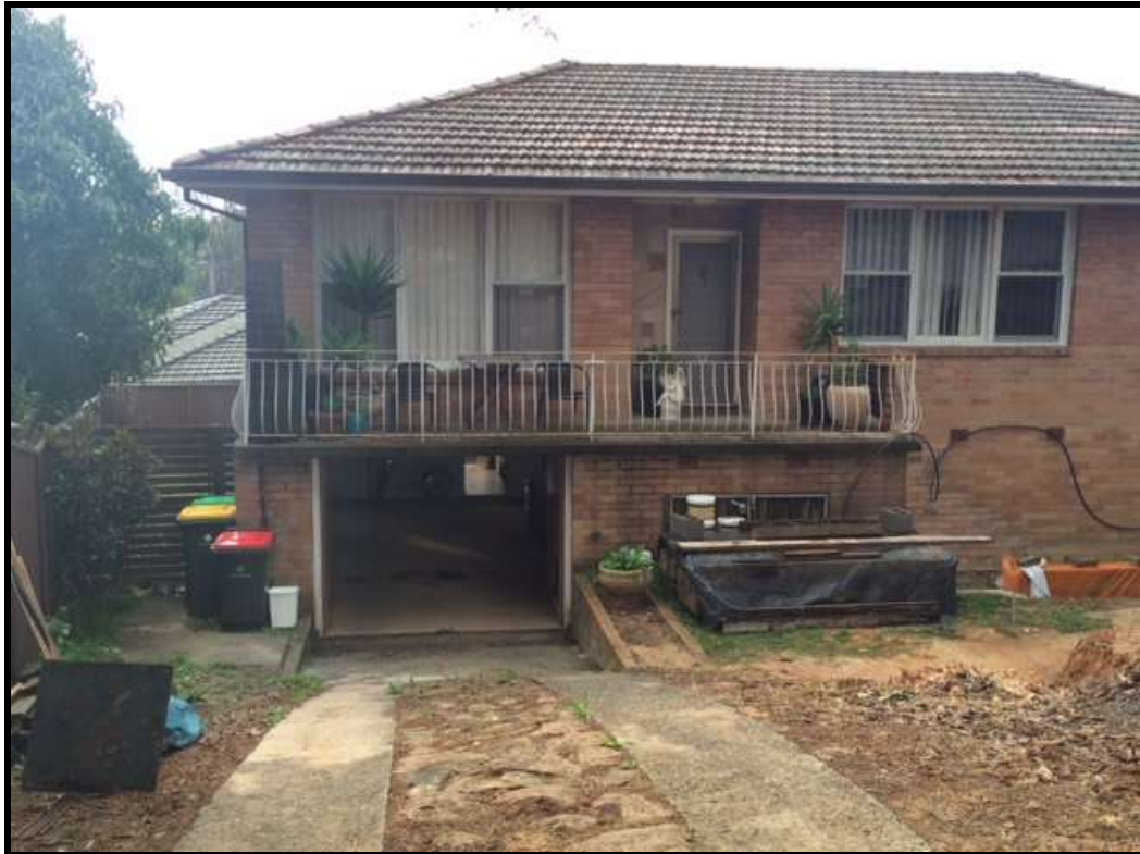
Figure 2 – View of subject site from the Conrad Street frontage. Noted in this image is the existing garage on the ground floor of the dwelling. Also noted is the existing front balcony which demonstrates a prevailing level of overlooking inherent to subject site and adjoining property at No.36 Conrad Street. Source: CPS photograph
