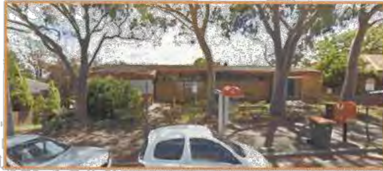
Figure 2 – Front of the existing building, No 176-178 Blaxland Road, Ryde (Source: googlemaps)
