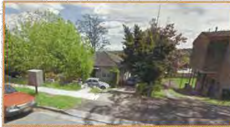
Figure 5 – View of existing single dwelling on southern side of rezoning site on Blaxland Road. (Source: googlemaps)
