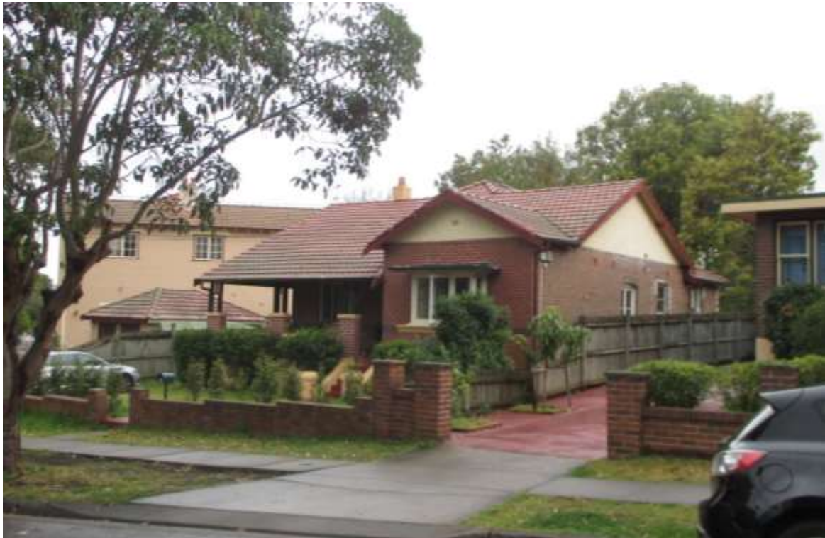
Figure 2. View of the site from Clive Road
