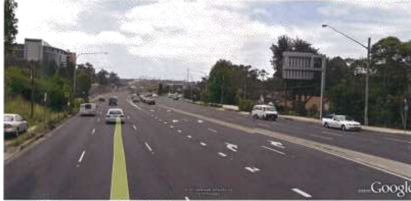
VIEW TO SOUTH
